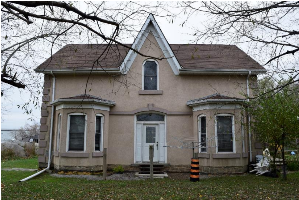
Image 2: Current front façade, note cut stone foundation and attempt to disguise a modern square headed window in the center gable.
