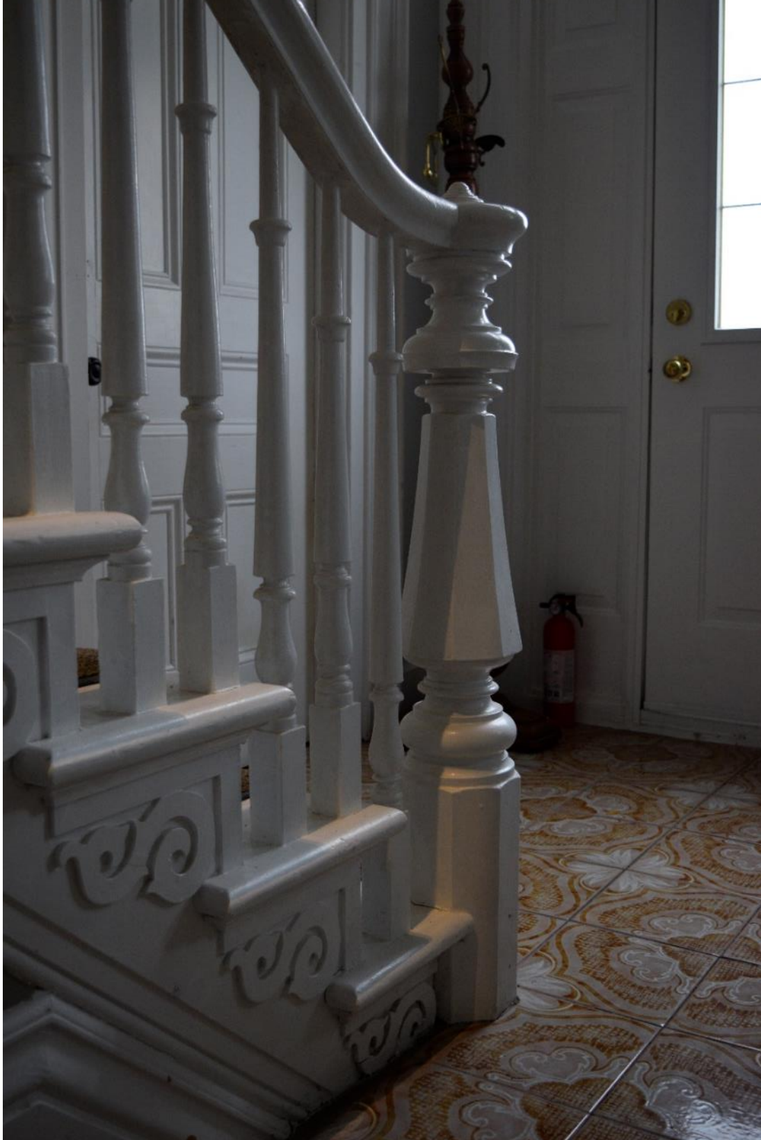
Image 18: Close up of original newel post, note non-original ceramic tile.
