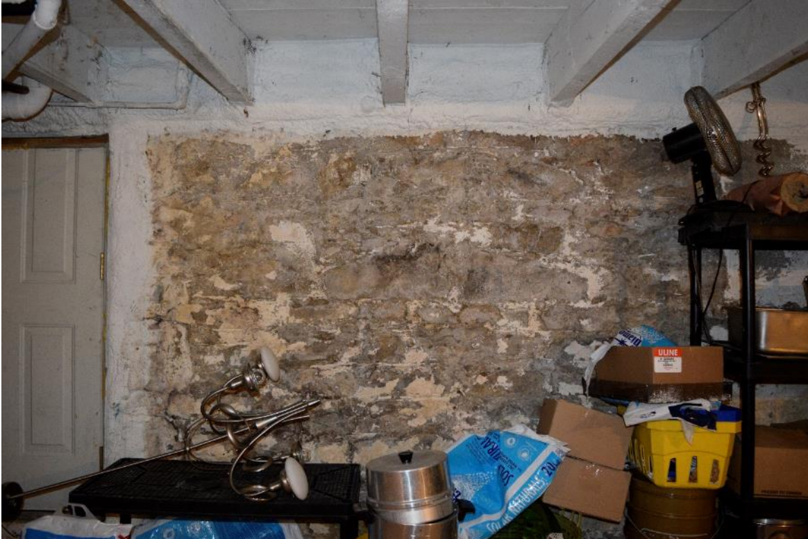
Image 26: Example of field stone foundation.
