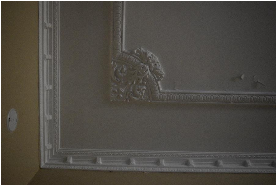
Image 24: Close up of c.1980 “chalk mouldings” used through the residence.
