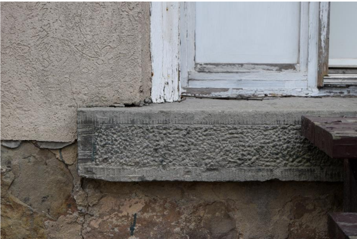
Image 7: Exposed cut stone threshold at front door.
