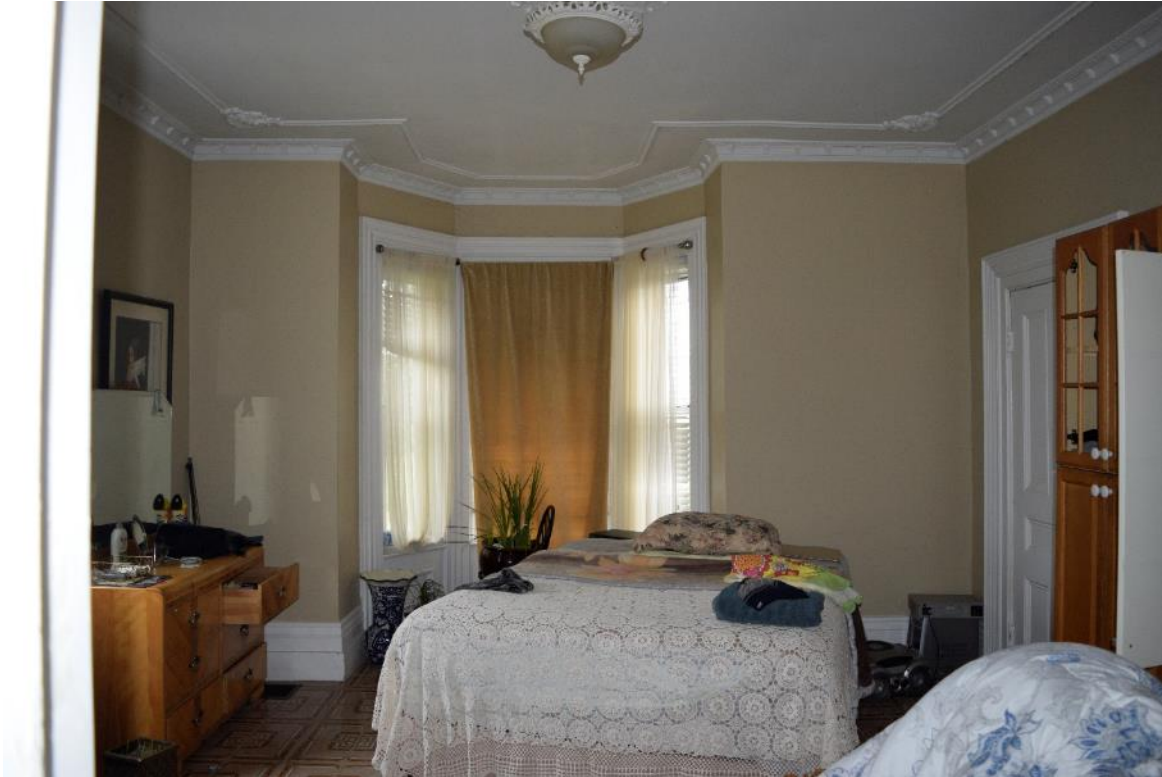
Image 23: Example of bay construction, note non-original “chalk mouldings” on ceiling.
