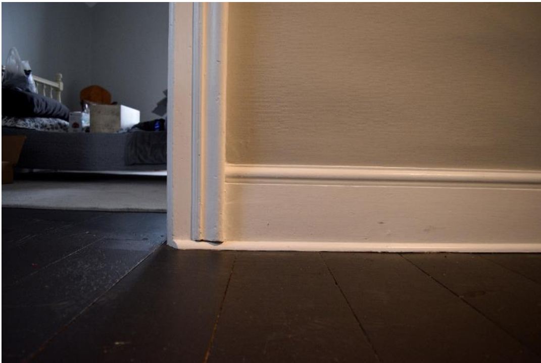
Image 13: Example of typical original baseboard and door trim on second floor.
