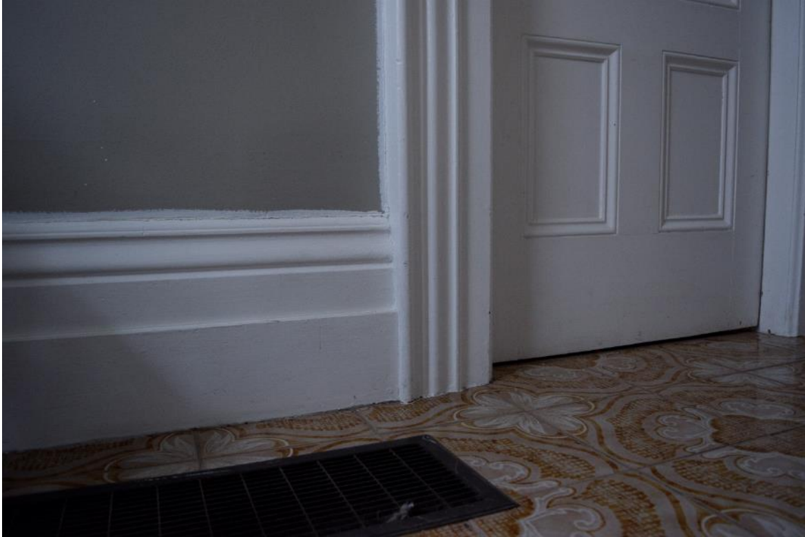
Image 14: Typical example of original baseboard and door trim on first floor.
