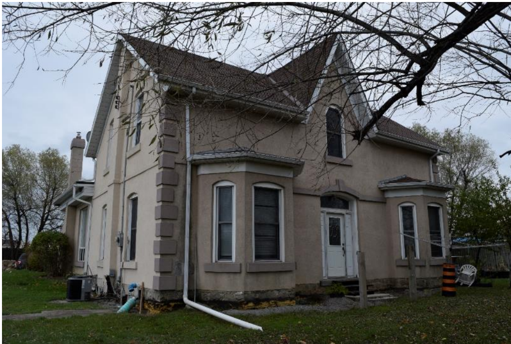
Image 3: Front and side view, note use of fake quoining at corner central belt containing key stone above main entrance.
