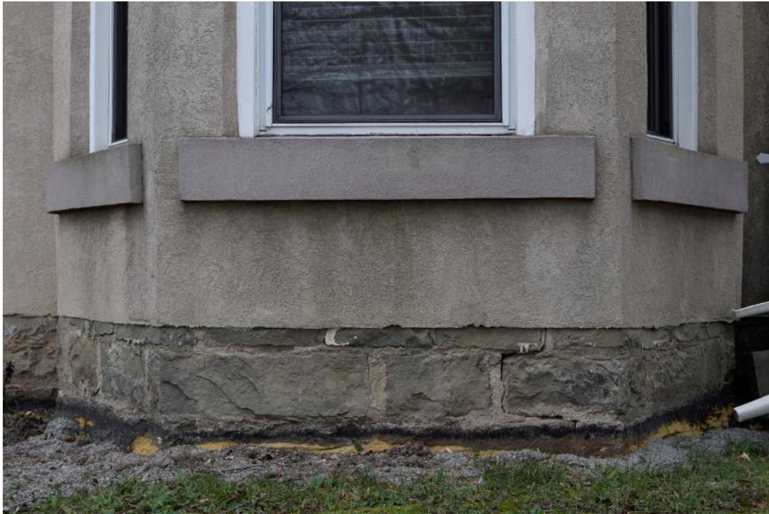
Image 8: Example of bay window, note evidence of spray-on waterproofing membrane on foundation stones, lug sills have been coated in stucco.
