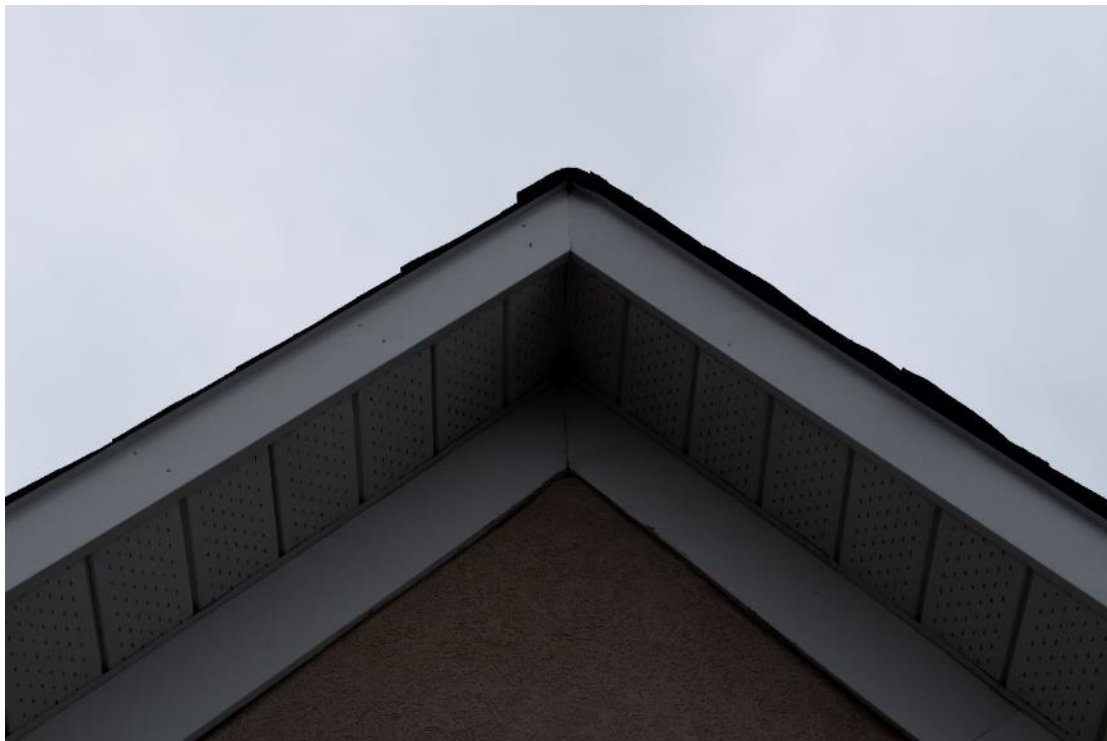
Image 9: Typical example of modern aluminum fascia, soffit and frieze.
