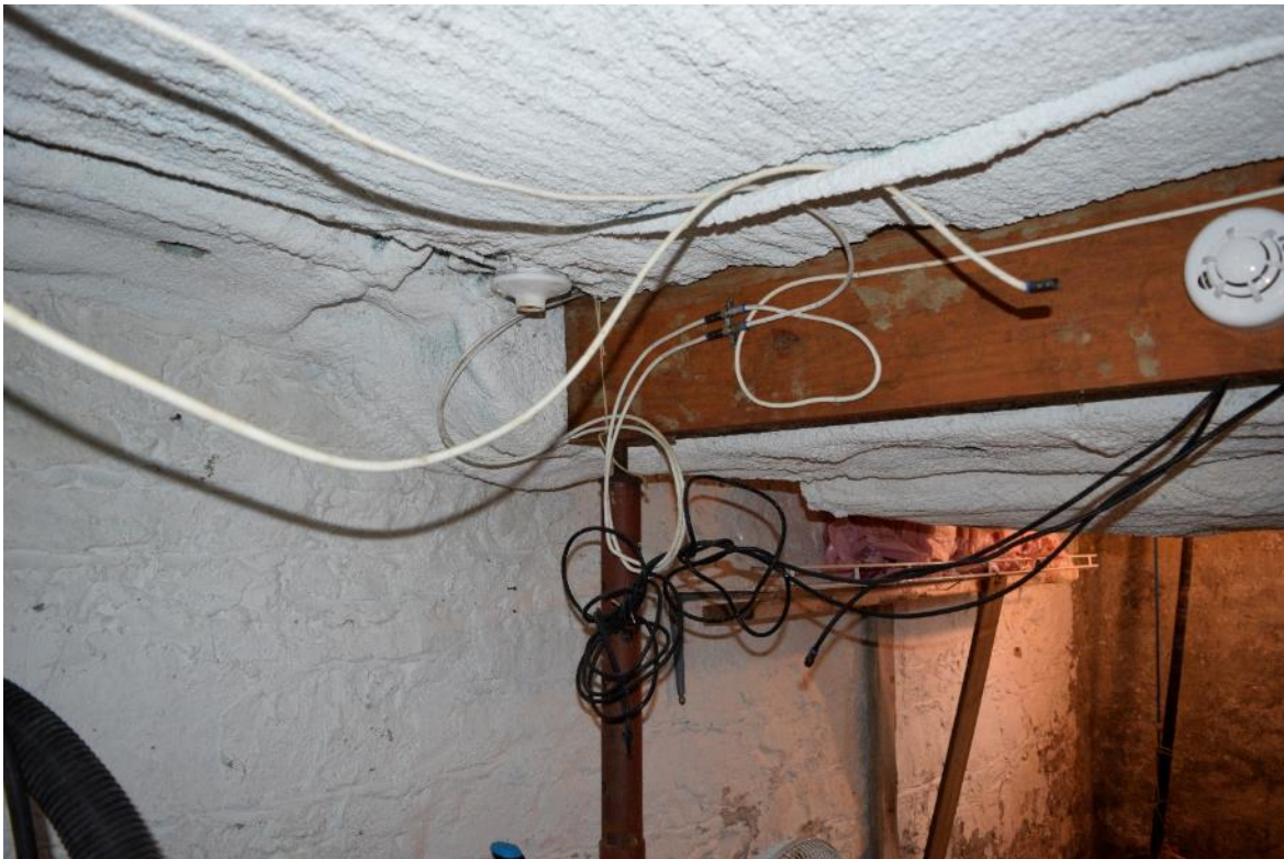
Image 27: Example of floor bracing and support posts used to augment floor joists of first floor.
