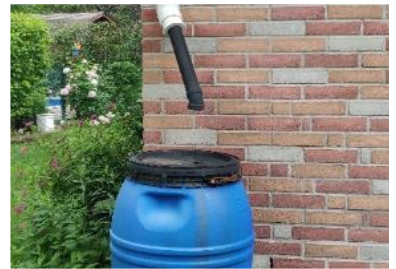
Many local residents are using rain barrels for rainwater harvesting. Photo Credit: CVC
