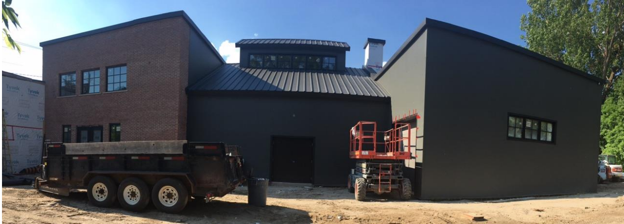
Furnace Room Brewery, 1 Elgin Street, August 2018 Photo Source: Furnace Room Brewery
