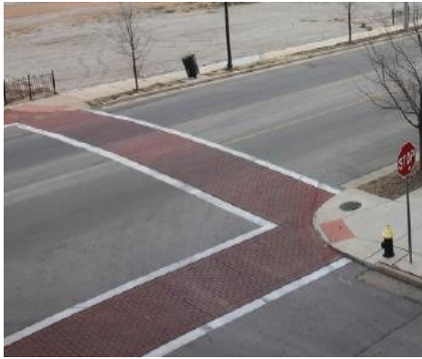
Figure 3: Example of Impressed Crosswalk
