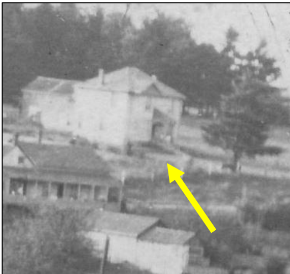
Figure 9: View of the subject property, c.1916 (EHS 10299)
