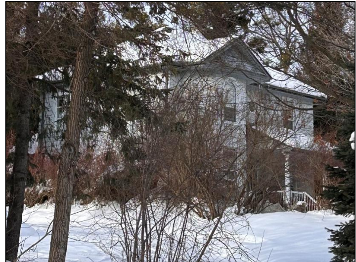
Figure 27: Obscured side (southwest) elevation of the subject property (Town of Halton Hills 2026)
