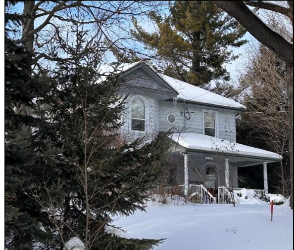
Figure 25: Front (southeast) elevation of the subject property (Town of Halton Hills 2026)
