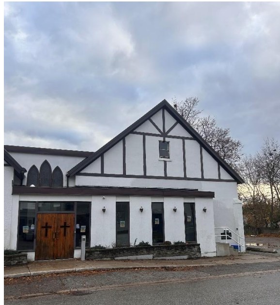
Figure 36: Partial northeast elevation of the existing building at 19 St. Alban's Drive (Town of Halton Hills 2025)
