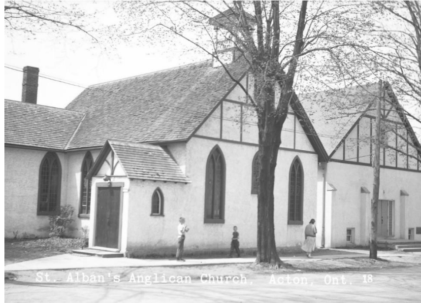
Figure 15: St. Alban the Martyr Anglican Church, c.1955, showing the newly constructed Parish Hall adjacent to the church (EHS 25068)
