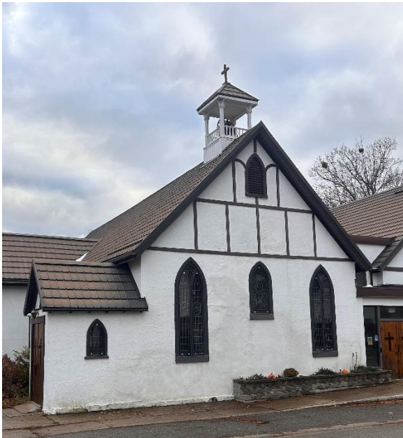
Figure 35: Partial northeast elevation of the existing building at 19 St. Alban's Drive (Town of Halton Hills 2025)
