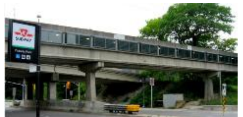
Figure 4 - Crescent Town Bridge, Toronto
