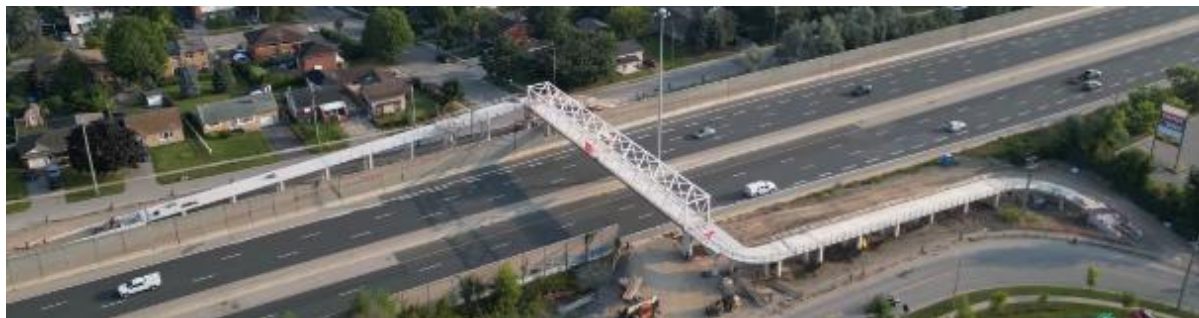
Figure 10 - Footprint of ramp connections for the new pedestrian and cycling bridge over Highway 7/8 in Waterloo Region, ON; Source: Region of Waterloo
