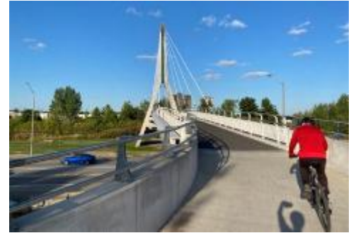
Figure 1 - Juno Beach Memorial Bridge, Ottawa
