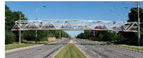
Figure 2 - Lake Wabukayne Trail Pedestrian Bridge, Mississauga
