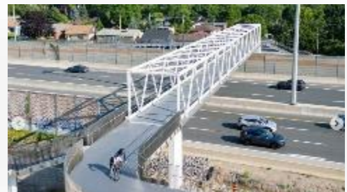
Figure 5 - Highway 7 / 8 Pedestrian Bridge, Kitchener
