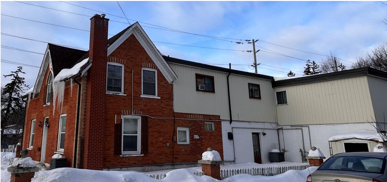
Figure 24: Southeast elevation of the Hamilton-Reed House and rear addition at 65 Main Street North (Town of Halton Hills 2026)
