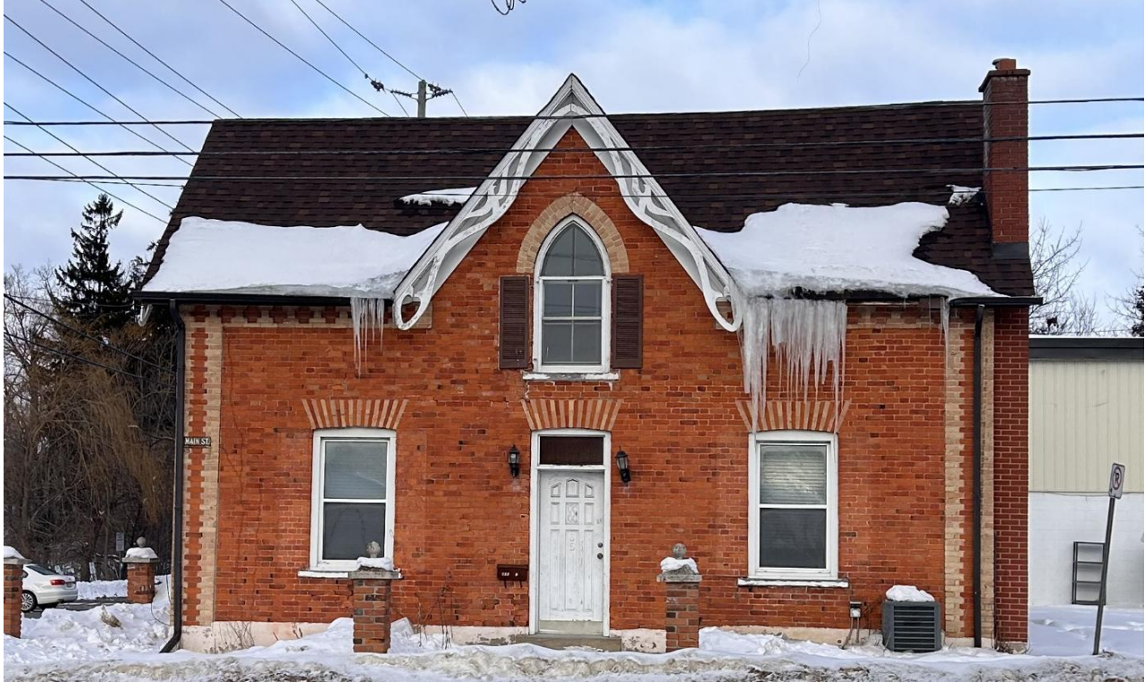
Hamilton-Reed House 65 Main Street North, Acton, Town of Halton Hills
