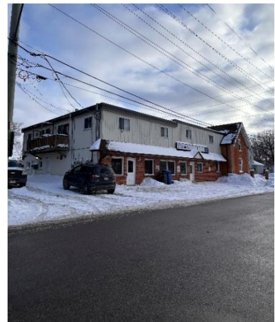
Figure 18: Looking southwest along River Street towards the subject property (Town of Halton Hills 2026)
