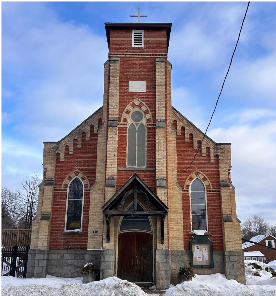
Figure 29: Front (northwest) elevation of the existing building at 64 Church Street East (Town of Halton Hills 2026)
