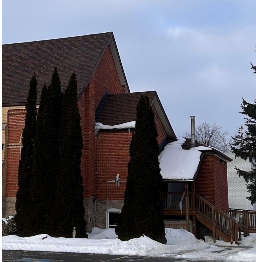
Figure 34: Rear (southeast) elevation and additions on the existing building at 64 Church Street East (Town of Halton Hills 2026)
