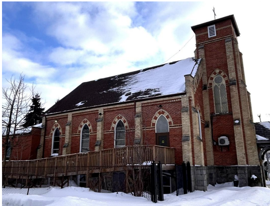
Figure 33: Side (northeast) elevation of the existing building at 64 Church Street East (Town of Halton Hills 2026)
