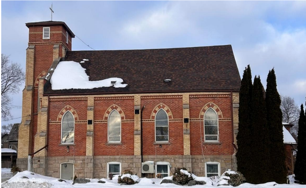
Figure 32: Side (southwest) elevation of the existing building at 64 Church Street East (Town of Halton Hills 2026)
