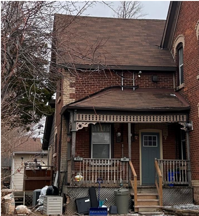
Figure 21: Front (southwest) elevation of the rear wing of the existing building at 49-51 Main Street North (Town of Halton Hills 2026)
