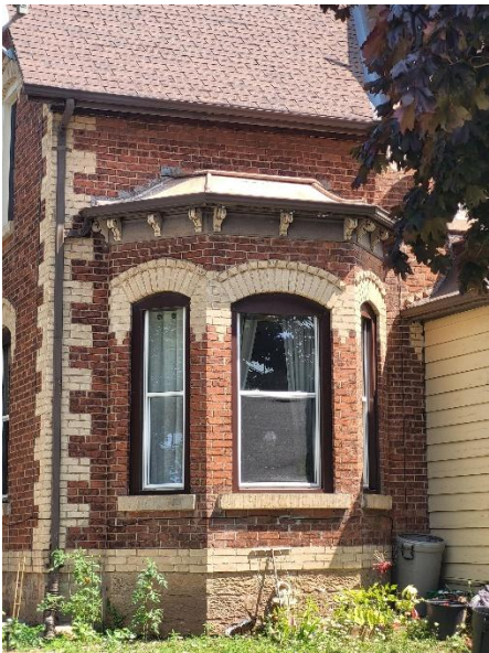
Figure 19: Detail of the projecting bay on the front (southwest) elevation of the existing building at 49-51 Main Street North (Town of Halton Hills 2025)
