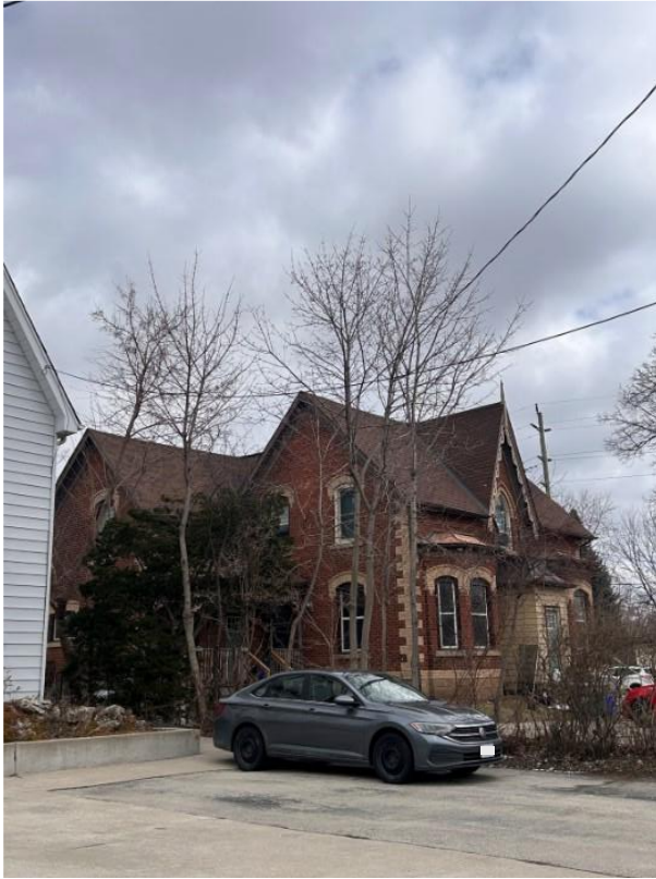
Figure 16: Looking west towards the subject property at the corner of Main Street North and Ewing Street (Town of Halton Hills 2026)
