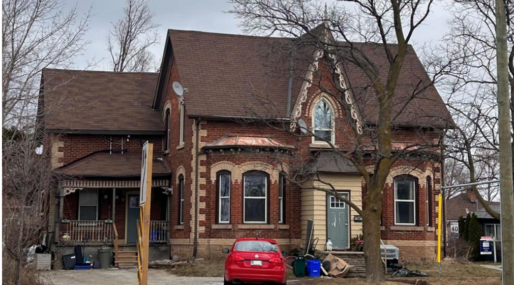
Figure 18: Front (southwest) elevation of the existing building at 49-51 Main Street North (Town of Halton Hills 2026)
