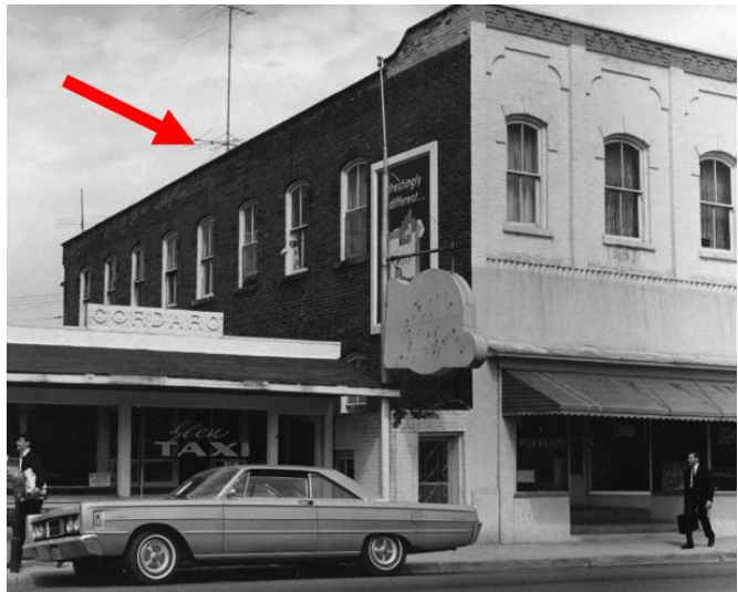
Figure 13: Creelman Factory Building identified along Main Street in Georgetown, c.1966 (EHS 17038)
