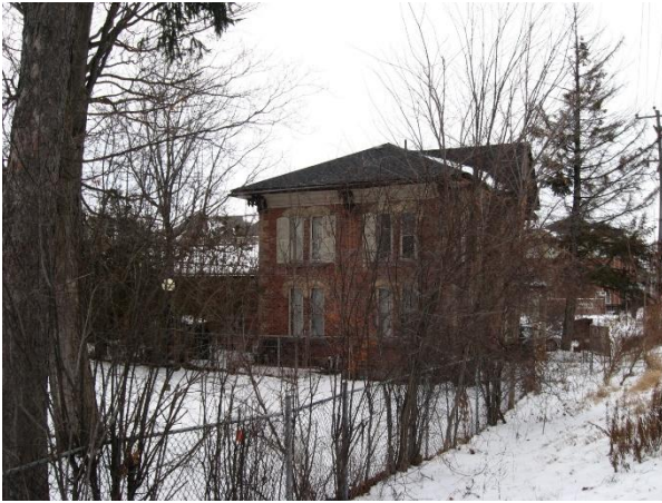
Figure 27: Moore-Creelman House, c.2016 (EHS 23169)
