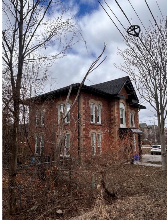
Figure 32: Looking northwest towards the subject property along Main Street North (Town of Halton Hills 2026)
