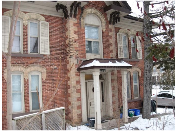
Figure 28: Detail of the front facade of Moore-Creelman House, c.2016 (EHS 23169)
