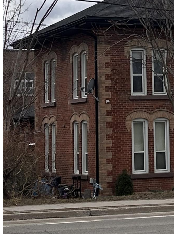
Figure 35: Looking towards the southeast elevation of the existing building at 44 Main Street North (Town of Halton Hills 2026)
