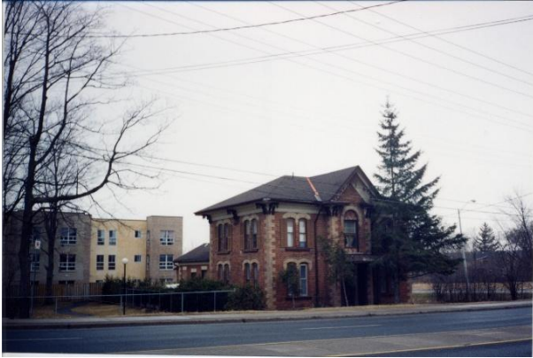
Figure 22: Moore-Creelman House, c.1995 (EHS 13164)
