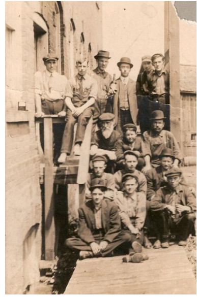
Figure 10: Workers on the steps of the Creelman Factory Building, c.1910 (EHS 20760)
