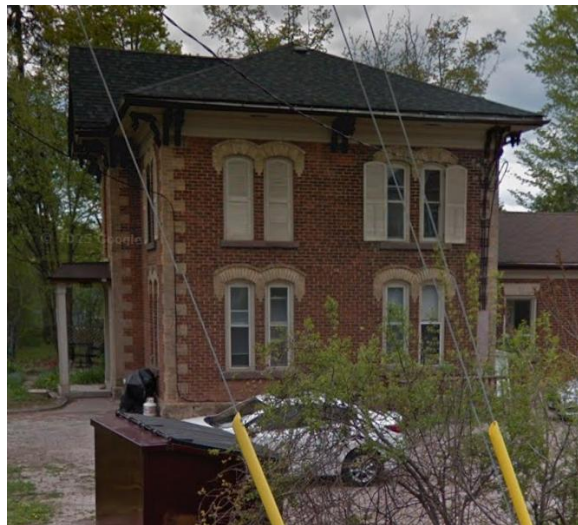
Figure 38: Google Streetview of the side elevation of the Moore-Creelman House (Google Streetview 2016)
