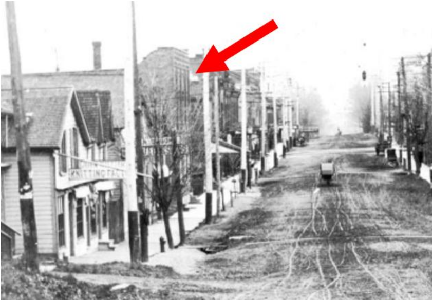
Figure 9: Creelman Factory Building along Main Street, Georgetown, c.1900 (EHS 26085)
