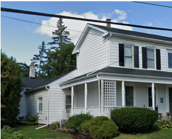
Figure 21: Side (south) elevation of the existing building at 508 Main Street (Town of Halton Hills 2025)
