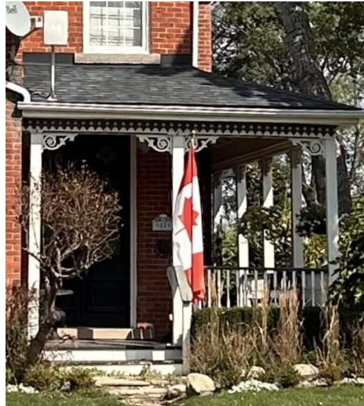
Figure 25: Front porch of the subject dwelling with decorative wooden frieze and brackets (Town of Halton Hills 2025)
