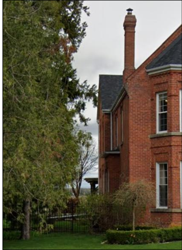
Figure 27: Partial side (northwest) elevation of the subject dwelling (Google Streetview 2022)
