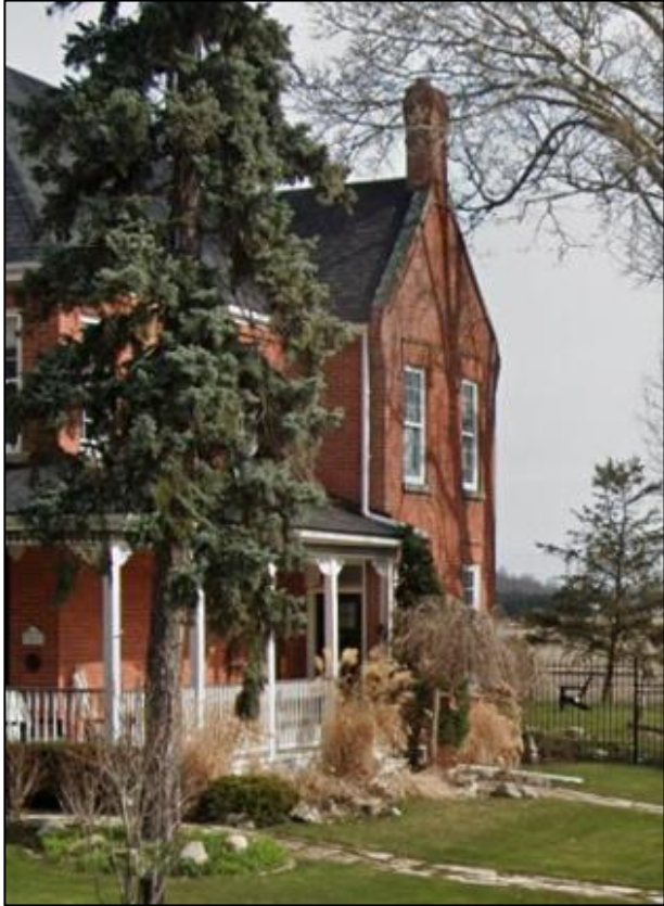
Figure 26: Partial side (southeast) elevation of the subject dwelling (Google Streetview 2022)
