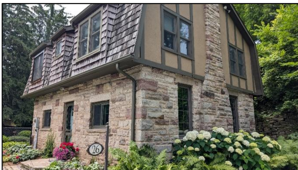
Figure 24: Partial front and side elevation of the subject property (J.M. Rowe 2024)
