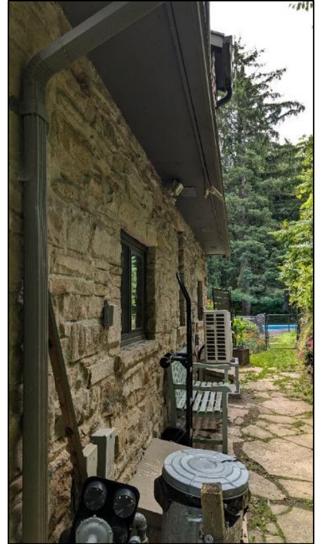
Figure 29: Rear (southwest) elevation of the subject property (J.M. Rowe 2024)
