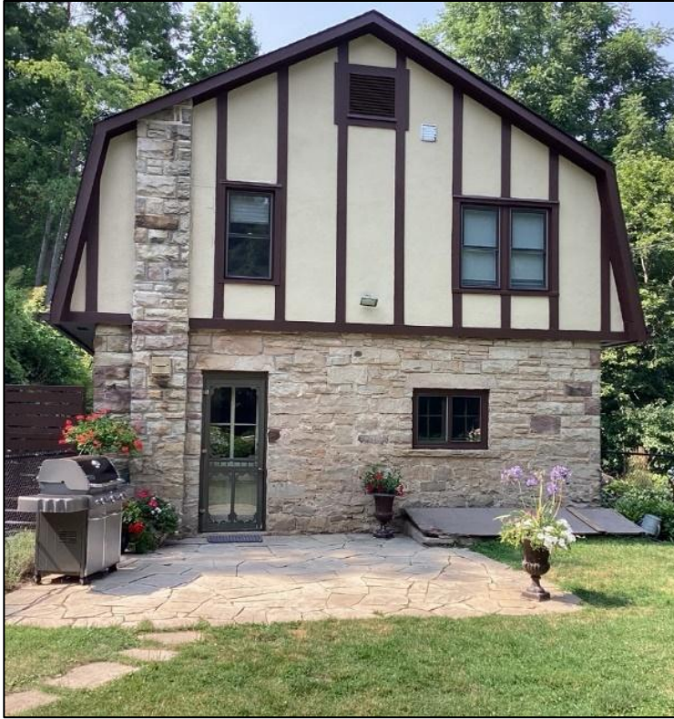
Figure 28: Side (southeast) elevation of the subject property (J.M. Rowe 2024)
