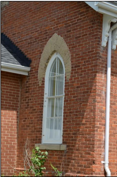
Figure 23: Lancet arched window with a buff brick hood mould and stone sill (Town of Halton Hills 2015)
