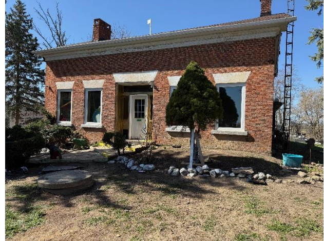
Figure 19: Front façade with significant alteration to front door, sidelights and transom and six over six windows.
