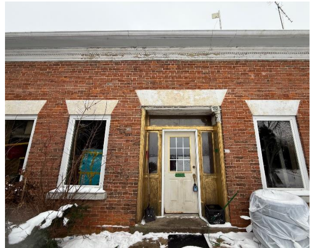
Figure 19: Front façade with significant alteration to front door, sidelights and transom and six over six windows.
