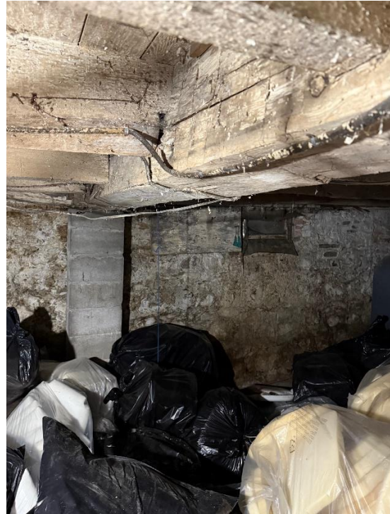
Figure 25: Basement foundation looks relatively stable with the original log beams. Minor water leakage was observed during the site visit.
