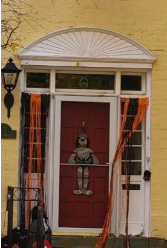
Figure 29: Front entry featuring sidelight windows, transom, and wooden sunburst pediment (Town of Halton Hills 2024)
