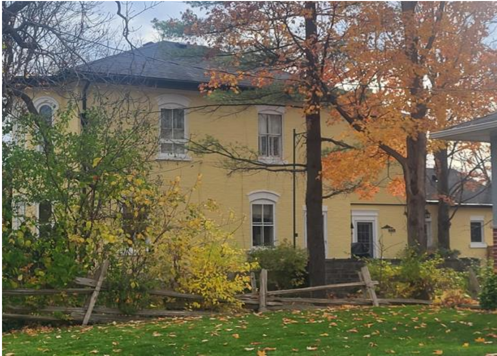
Figure 35: Side (northwest) elevation (Town of Halton Hills 2024)
