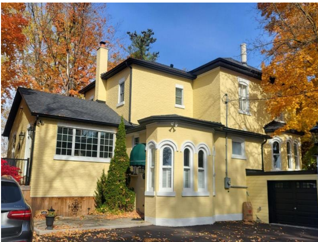
Figure 31: Side (southeast) elevation (Town of Halton Hills 2024)
