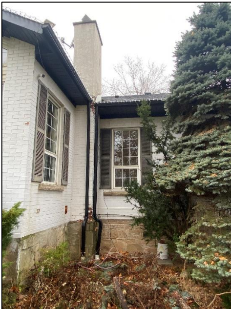
Figure 34: Side (southeast) elevation of the subject dwelling (Town of Halton Hills 2024)
