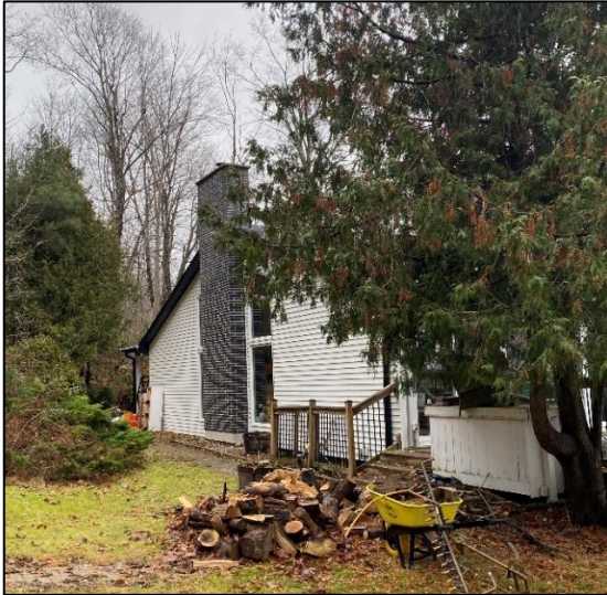
Figure 36: Rear (southwest) elevation of the subject dwelling (Town of Halton Hills 2024)
