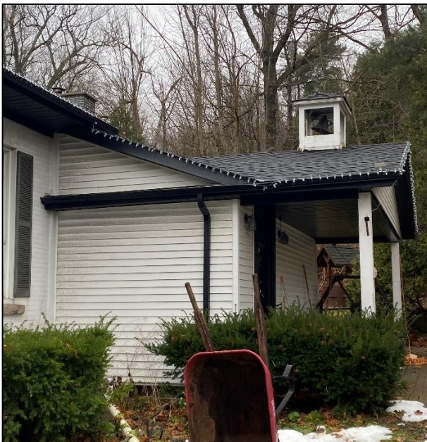
Figure 30: Contemporary addition on the subject dwelling (Town of Halton Hills 2024)
