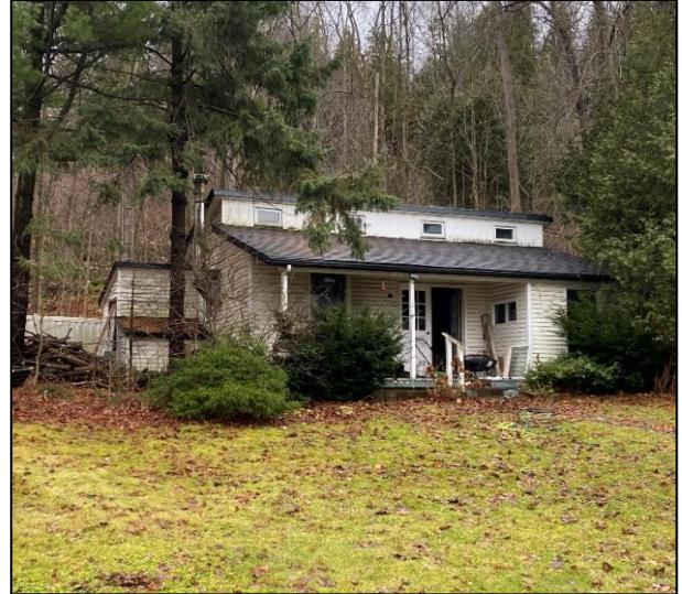
Figure 37: Rear contemporary accessory structure (Town of Halton Hills 2024)
