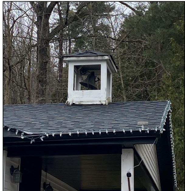
Figure 31: Bell and cupola located on the roof of the contemporary addition (Town of Halton Hills 2024)
