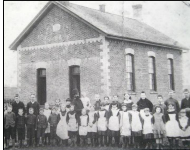
Figure 47: Former Zion School, S.S. No. 12, built c.1869, photograph taken c. 1890 (North York Historical Society)
