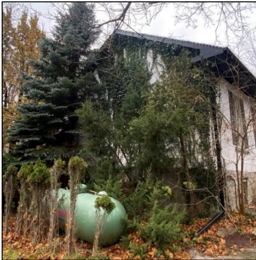
Figure 26: Front (northeast) elevation obscured by vegetation (Town of Halton Hills 2024)
