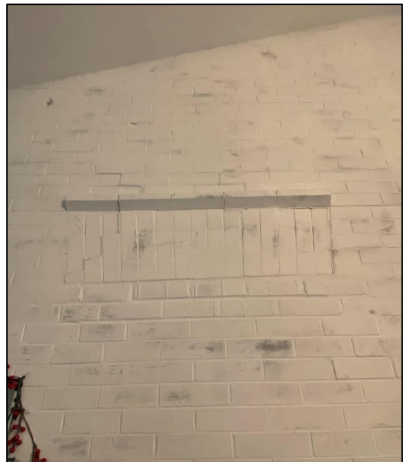
Figure 39: Brick soldier course lintel located above the former entryway (Town of Halton Hills 2024)
