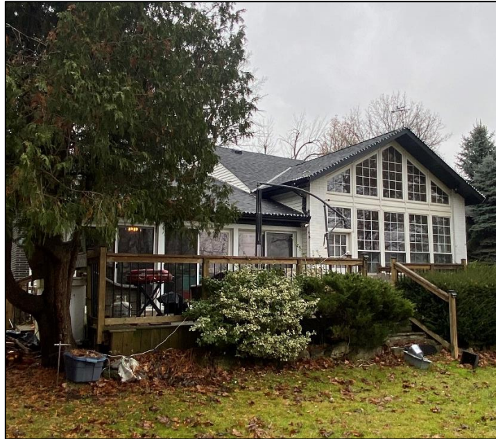
Figure 35: Side (southeast) elevation of the subject dwelling showcasing the contemporary addition (Town of Halton Hills 2024)
