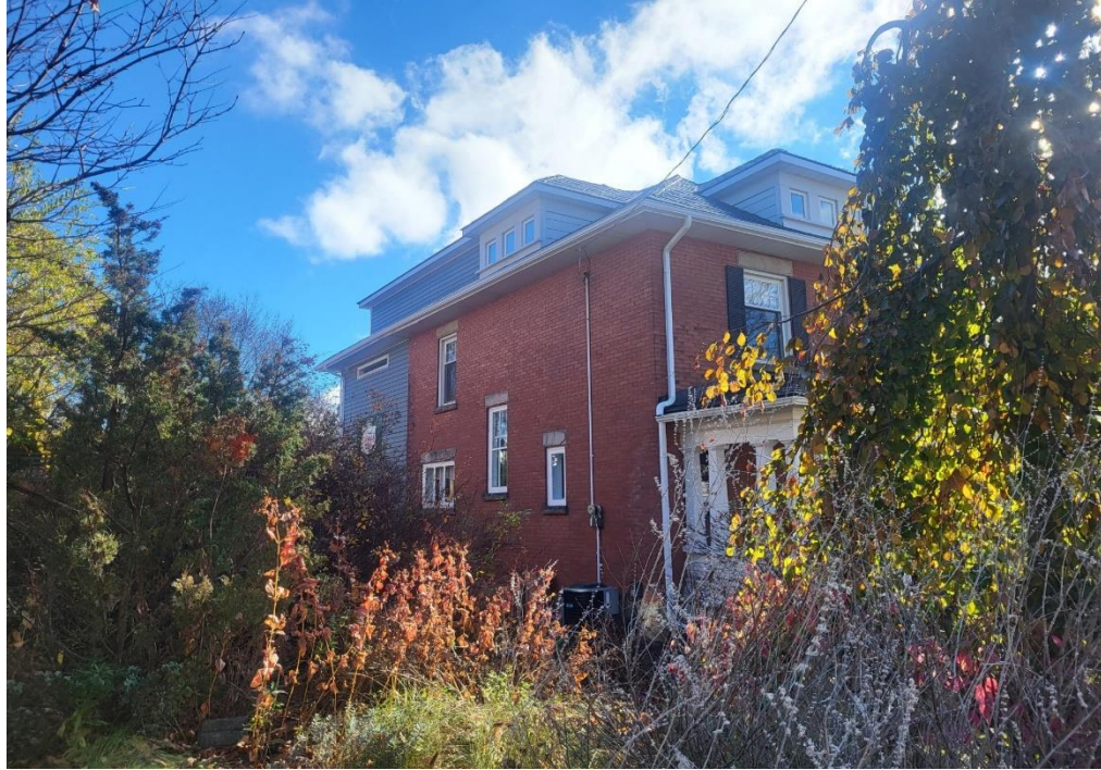
Figure 22: Side (northeast) elevation (Town of Halton Hills 2024)
