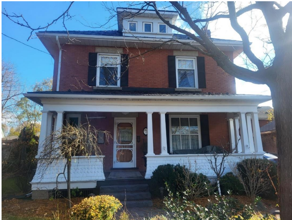
Figure 18: Front (northwest) Elevation (Town of Halton Hills 2024)
