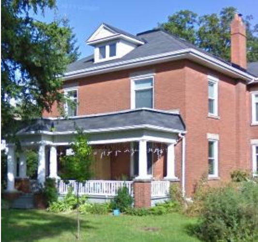
Figure 27: Edwardian style home located at 4 King Street (Google Streetview 2017)
