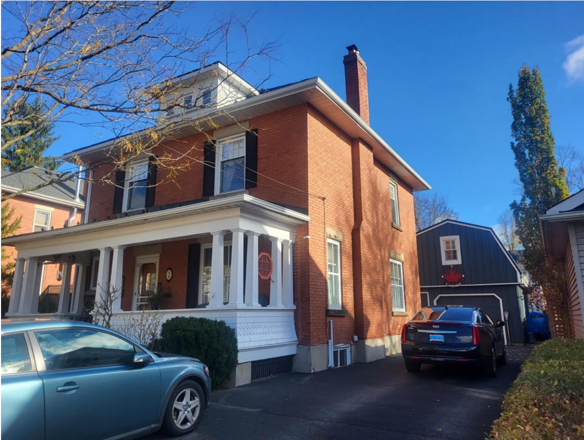
Figure 21: Obstructed partial side (southwest) elevation of the existing dwelling (Town of Halton Hills 2024)
