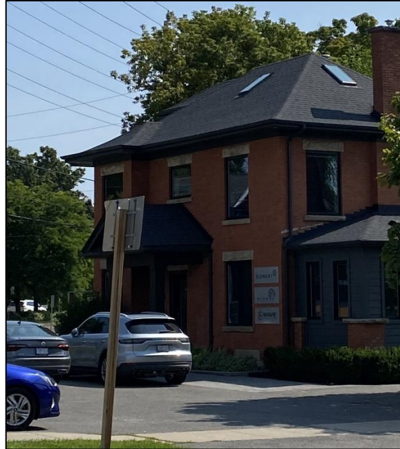
Figure 37: Front elevation of the subject building (Town of Halton Hills 2024)
