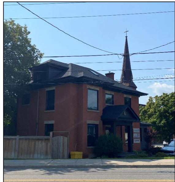
Figure 35: Front (northwest) elevation of the subject building (Town of Halton Hills 2024)
