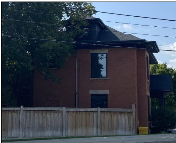
Figure 38: Side (northeast) elevation of the subject building (Town of Halton Hills 2024)
