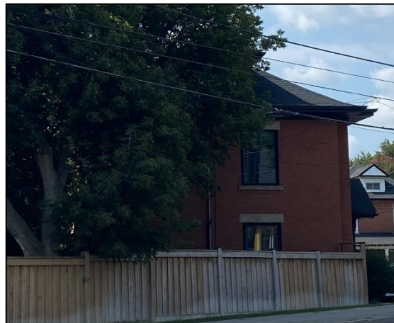
Figure 39: Partial side (northeast) elevation of the subject building obscured by vegetation (Town of Halton Hills 2024)
