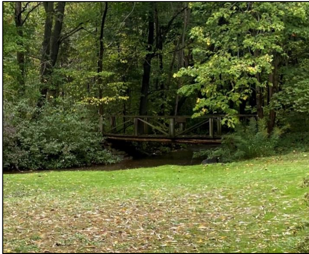
Figure 45: Wooden bridge spanning Silver Creek towards the rear of the property (Town of Halton Hills 2024)
