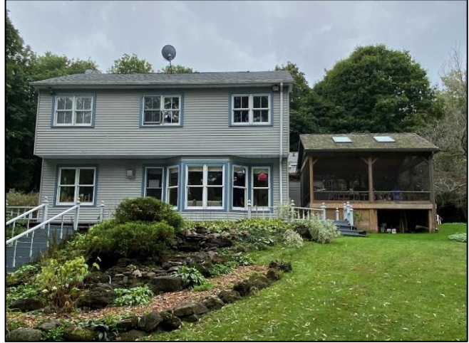
Figure 40: Rear (northeast) elevation of the subject dwelling (Town of Halton Hills 2024)
