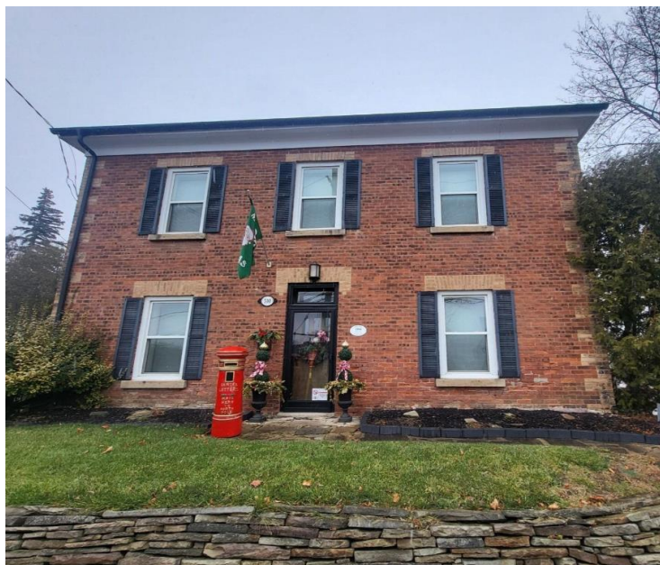
Figure 34: Front (southeast) elevation of the existing building at 510 Main Street Front (Town of Halton Hills 2024)
