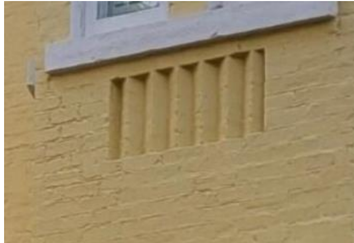
Figure 28: Inset "dogtooth" brick detailing on the projecting bay of 53 Charles Street (Town of Halton Hills 2024)
