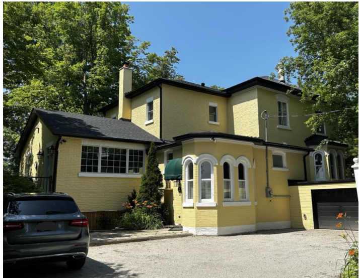
Figure 34: Side (southeast) elevation (Town of Halton Hills 2024)
