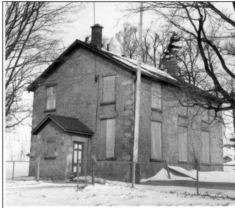
Figure 24: Gibraltar boarded up after closing and the opening of Limehouse, c.1962 (EHS 10318)
