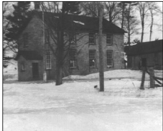
Figure 16: Exterior of Gibraltar Schoolhouse, c.1944 (EHS 11520)
