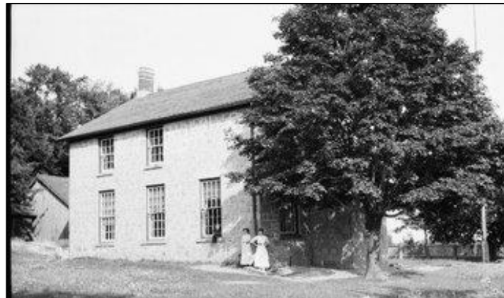
Figure 8: Exterior of Gibraltar Schoolhouse, c.1909 (EHS 19964)
