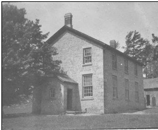
Figure 7: Exterior of Gibraltar Schoolhouse, c.1909 (EHS 21866)
