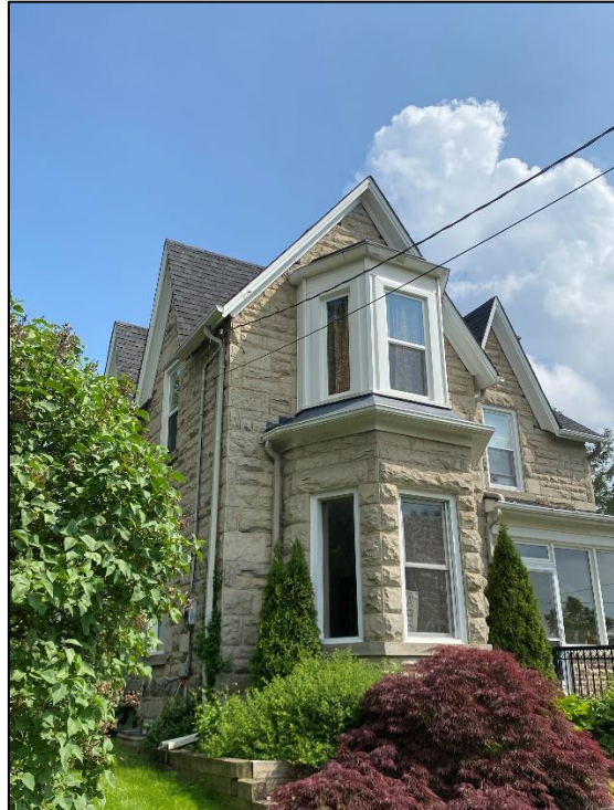
Figure 20: North corner of the existing dwelling (Town of Halton Hills, 2024)
