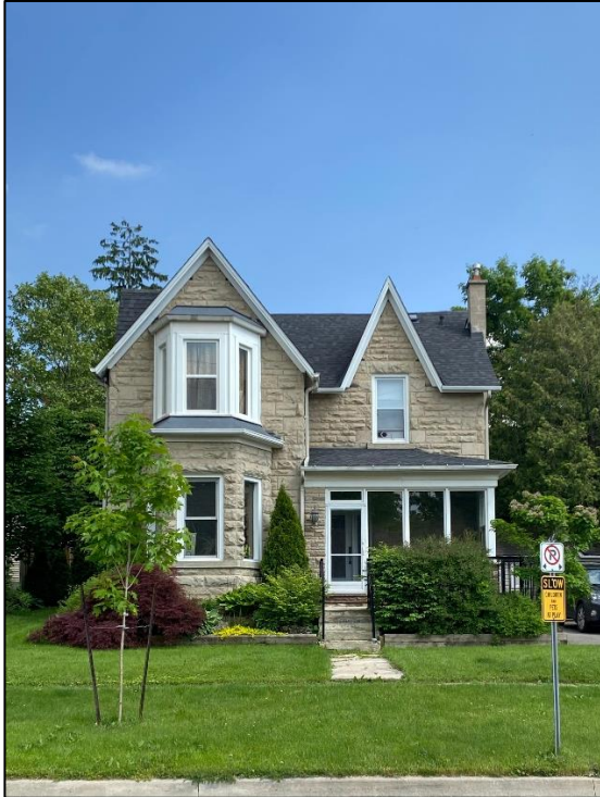
Figure 19: Front (northwest) elevation of the existing dwelling (Town of Halton Hills, 2024)
