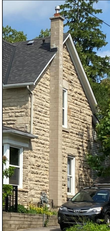
Figure 28: Side (southwest) elevation of the existing dwelling (Town of Halton Hills 2024)
