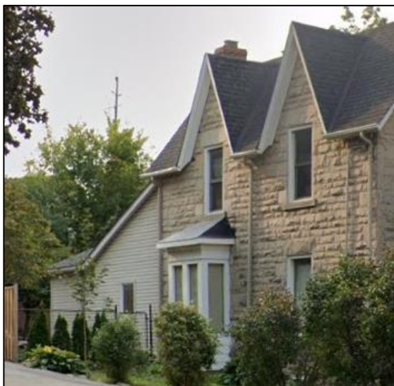
Figure 25: Side (northwest) elevation of the existing dwelling (Google Streetview 2020)
