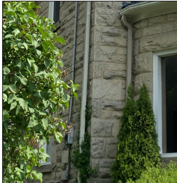
Figure 24: Staggered stone quoining along the front (northwest) elevation (Town of Halton Hills 2024)
