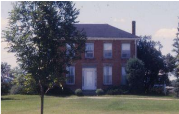
Figure 9: The subject property at 10295 10 Side Road c.1990s (EHS 18311).
