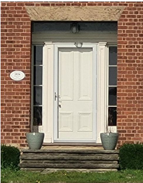
Figure 13: 10295 10 Side Road Entrance (Town of Halton Hills 2024)
