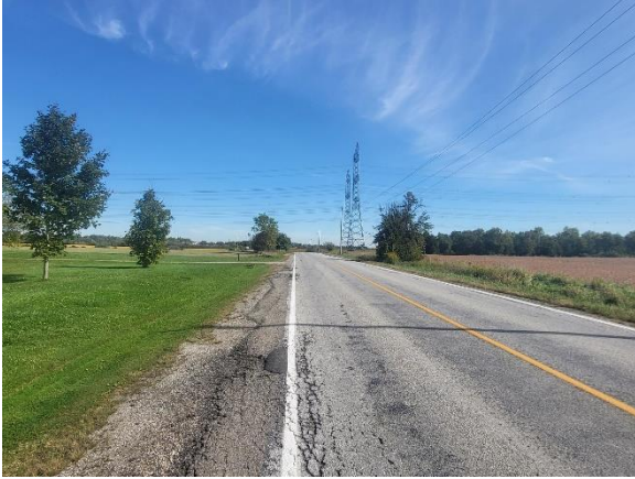
Figure 20: Looking northeast from the subject property (Town of Halton Hills 2024)
