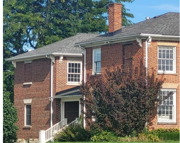
Figure 16: 10295 10 Side Road Side (southwest) Elevation (Town of Halton Hills 2024)
