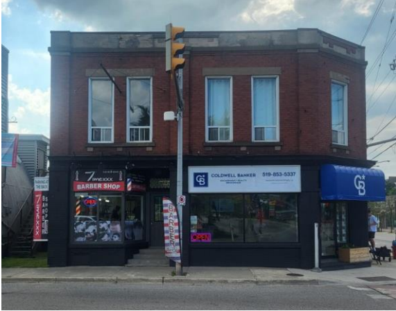
Figure 35: Northwest elevation of the existing building within the subject property (Town of Halton Hills 2024)
