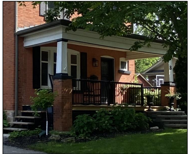
Figure 33: Existing covered wooden porch along the front (southwest) elevation (Town of Halton Hills 2024)
