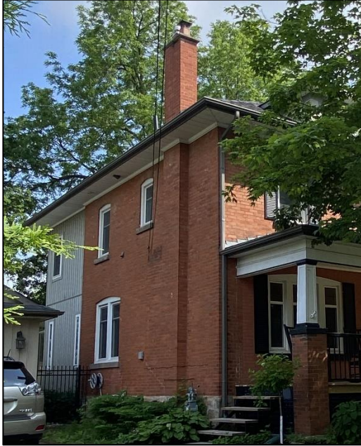
Figure 34: Side (northeast) elevation of the existing dwelling (Town of Halton Hills 2024)
