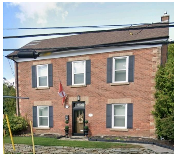
Figure 31: A Georgian Residence at 510 Main Street, Glen Williams. (Google Street View 2023)
