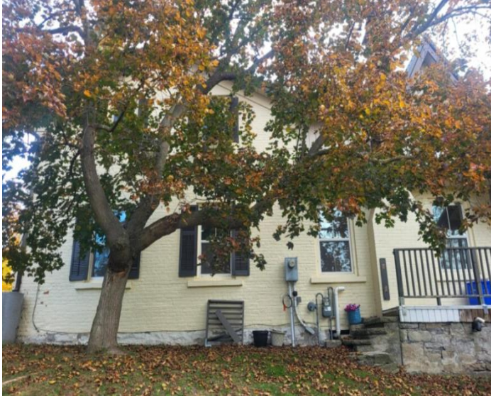
Figure 23: Side (southwest) elevation of the existing building at the subject property, slightly obscured by mature tree (Town of Halton Hills 2024)
