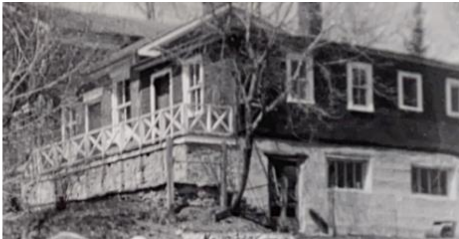
Figure 9: A 1956 photograph of the c.1920s-1930s rear addition constructed by the Thompson family (Courtesy of Christine Earl, 2024)
