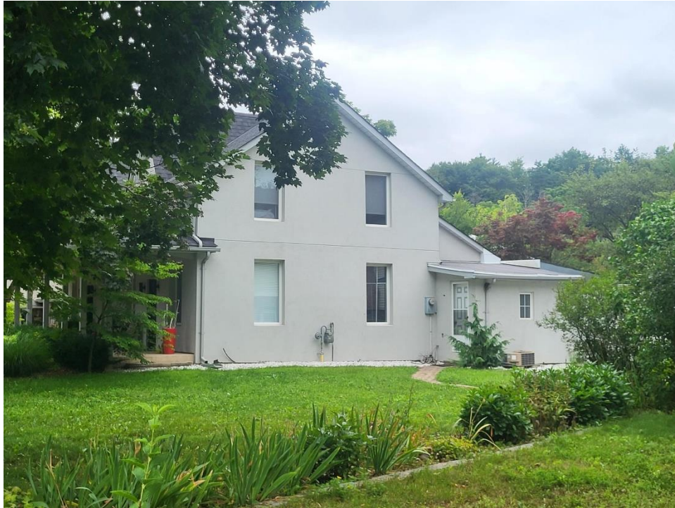
Figure 25: Side (south) elevation of the existing building at 12 & 14 Adamson Street North (Town of Halton Hills 2024)
