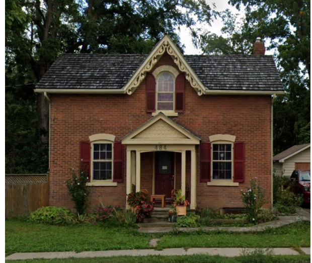
Figure 30: 484 Guelph Street, Norval (Google Street View 2023)
