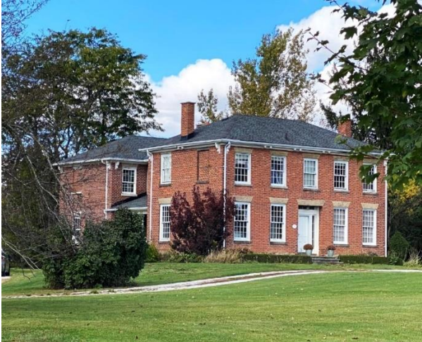
Figure 15: 10295 10 Side Road Side (southwest) Elevation (Town of Halton Hills 2024)
