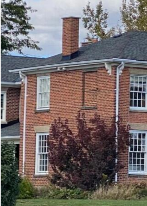
Figure 17: 10295 10 Side Road Side (southwest) Elevation (Town of Halton Hills 2024)
