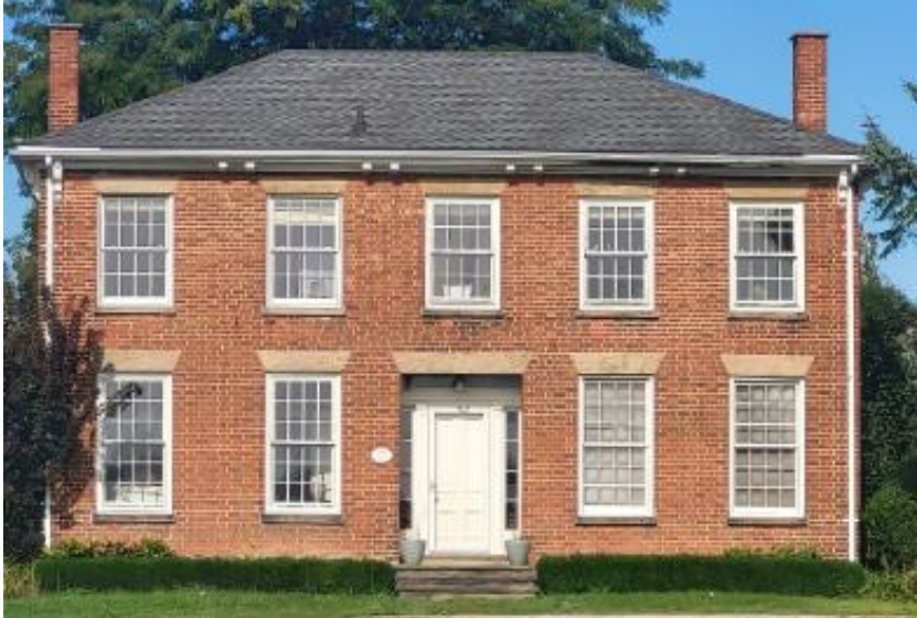
Figure 12: 10295 10 Side Road Front (southeast) Elevation (Town of Halton Hills 2024)
