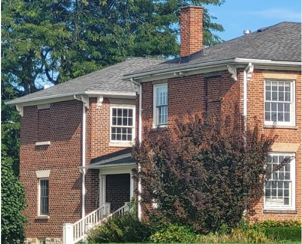
Figure 16: 10295 10 Side Road Side (southwest) Elevation (Town of Halton Hills 2024)
