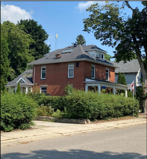
Figure 25: Side (southwest) elevation of the existing dwelling (Town of Halton Hills 2024)
