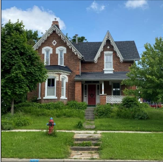
Figure 21: Front (northwest) elevation of the existing dwelling (Town of Halton Hills 2024)
