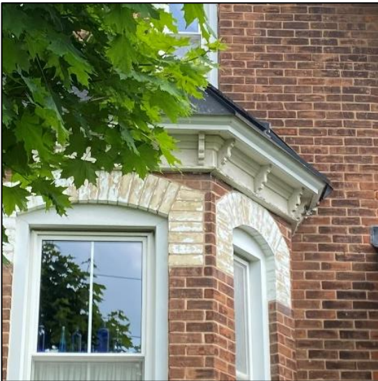
Figure 31: White paint weathering off the existing brick voussoirs (Town of Halton Hills 2024)
