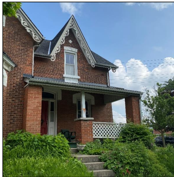
Figure 24: Front (northwest) elevation (Town of Halton Hills 2024)
