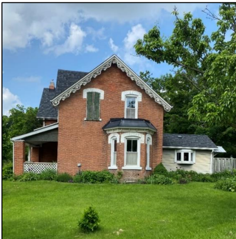
Figure 27: Side (southwest) elevation of the existing dwelling (Town of Halton Hills 2024)
