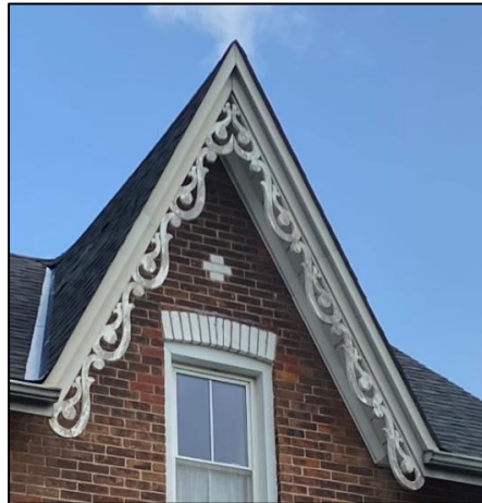
Figure 26: Decorative white brick in a cross pattern above the porch on the front (northwest) elevation (Town of Halton Hills 2024)
