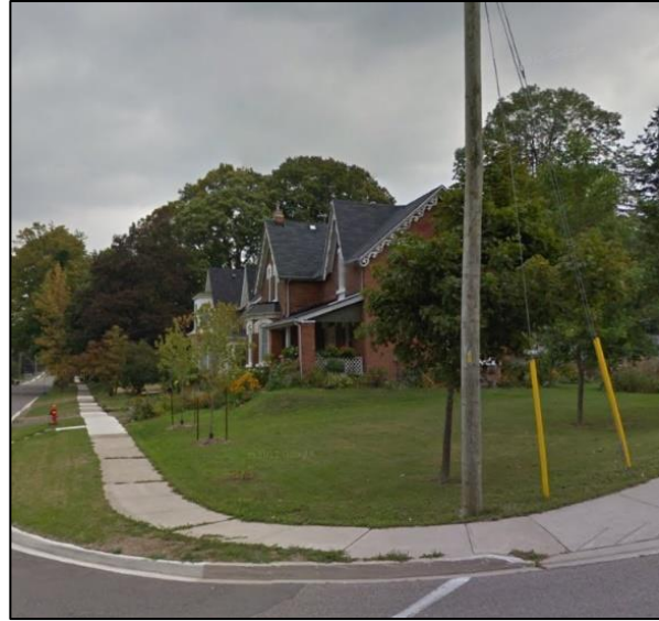
Figure 22: Looking towards Queen Street, viewing the partial front (northwest) and side (southwest) elevation (Google Streetview 2011)
