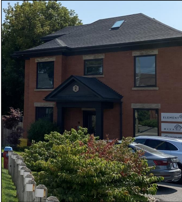
Figure 30: Front elevation of the subject building (Town of Halton Hills 2024)
