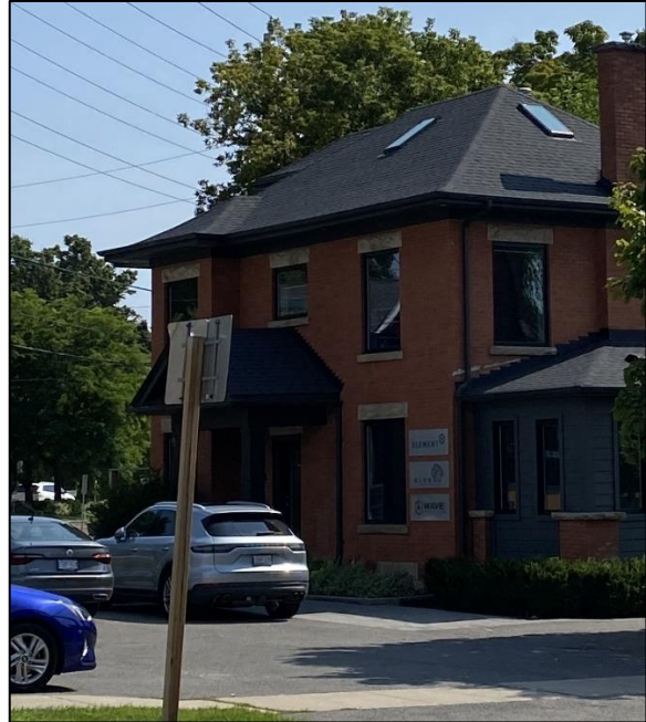
Figure 31: Front elevation of the subject building (Town of Halton Hills 2024)
