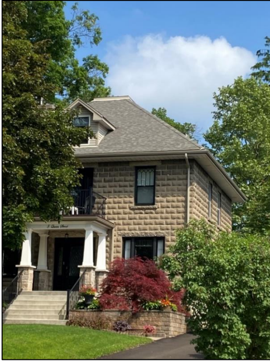
Figure 21: Partial front (northwest) elevation of the subject dwelling (Town of Halton Hills 2024)
