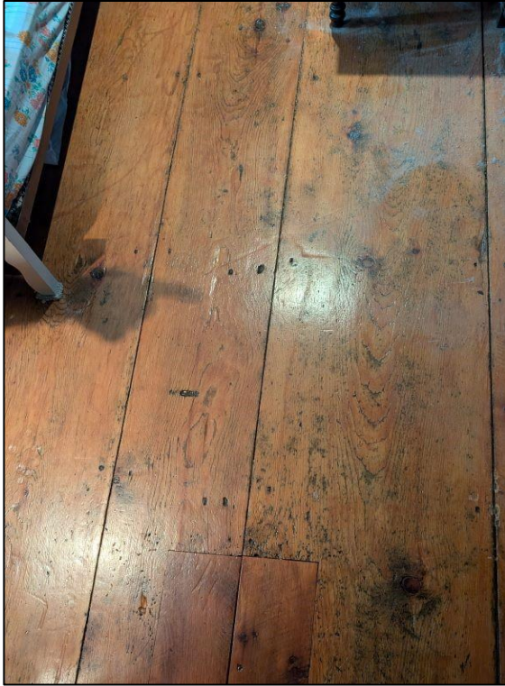
Figure 33: Existing pine floorboards found throughout the interior (John Mark Rowe 2024)
