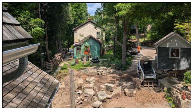
Figure 32: Rear (south) elevation of the subject dwelling (John Mark Rowe 2024)
