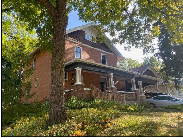
Figure 25: Partial front (northwest) elevation of the existing dwelling (Town of Halton Hills 2023)
