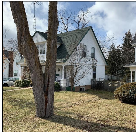
Figure 26: Partial side (northeast) elevation (Town of Halton Hills 2023)
