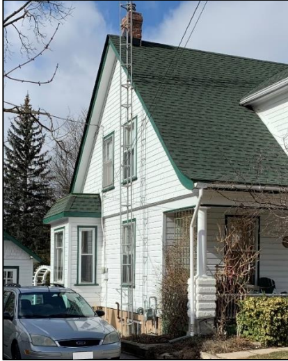
Figure 23: Partial side (southwest) elevation (Town of Halton Hills 2023)
