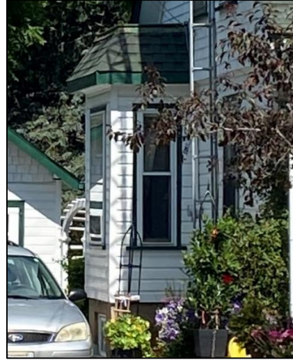
Figure 24: Partial view of the bay window along the side (southwest) elevation (Town of Halton Hills 2024)
