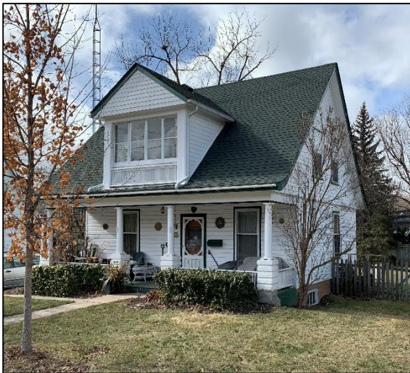
Figure 25: Partial side (northeast) elevation (Town of Halton Hills 2023)
