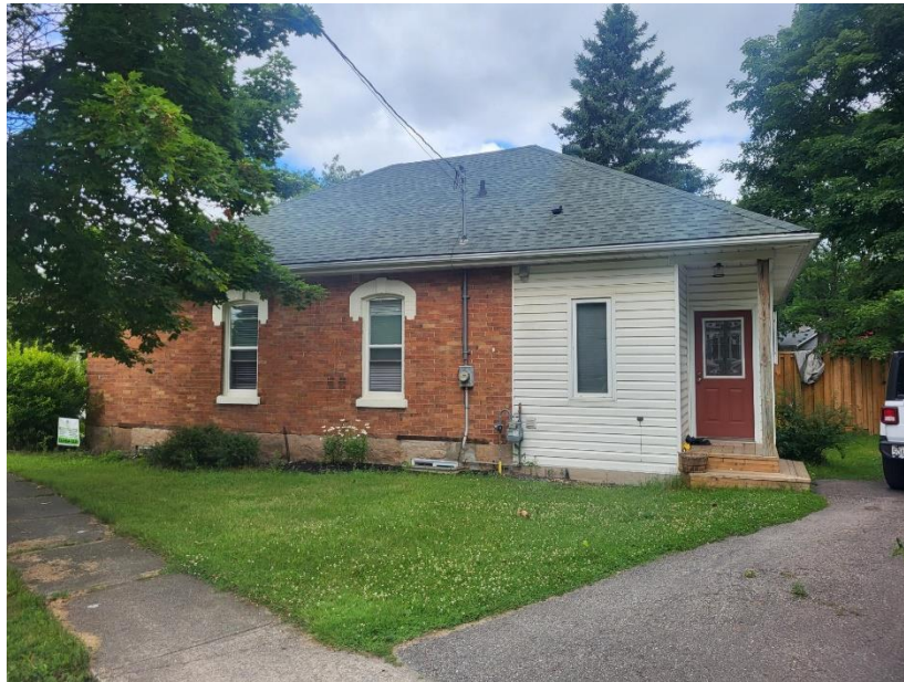
Figure 12: 23 Young Street, Side (East Elevation (Town of Halton Hills 2024)
