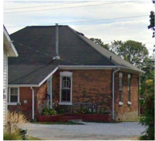
Figure 15: 56 Young Street, rear Elevation. (Town of Halton Hills, 2024).
