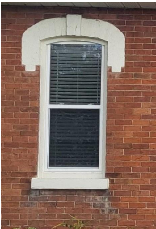
Figure 18: Window Detailing on 23 Young Street. (Town of Halton Hills, 2024).
