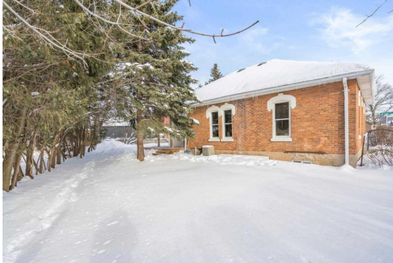
Figure 13: 23 Young Street, Side (West) Elevation (House Sigma 2023)
