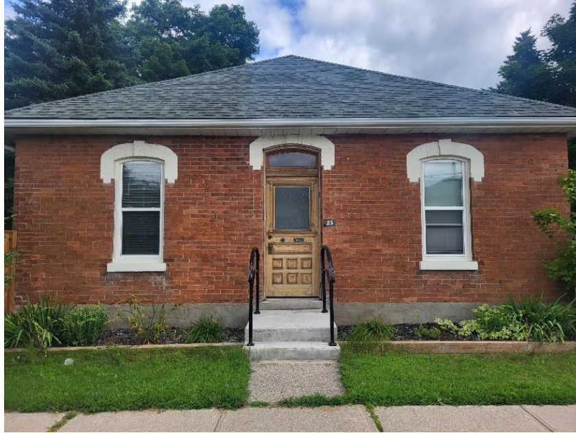
Figure 10: 23 Young Street, Front (South) Elevation (Town of Halton Hills 2024)
