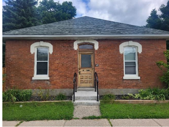
Figure 7: The front elevation of 23 Young Street in July 2024 (Town of Halton Hills 2024).
