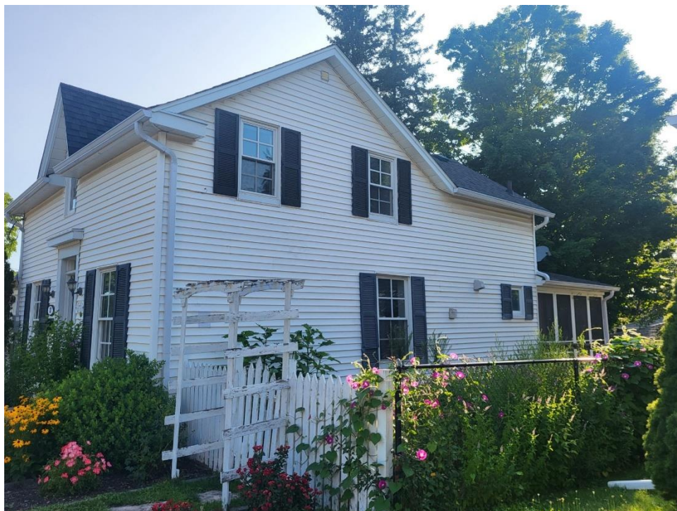
Figure 20: Side (south) elevation of the existing building at 12 Chapel Street (Town of Halton Hills 2024)
