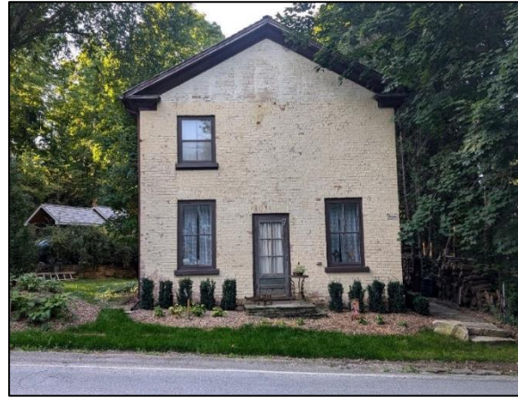
Figure 26: Side (north) elevation of the existing dwelling, fronting Prince Street (John Mark Rowe 2024)
