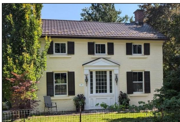
Figure 40: Example of a Georgian House at 15 Mountain Street, Glen Williams (John Mark Rowe 2024)
