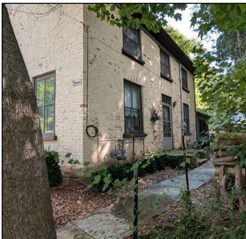
Figure 27: Front (west) elevation of the existing dwelling (John Mark Rowe 2024)
