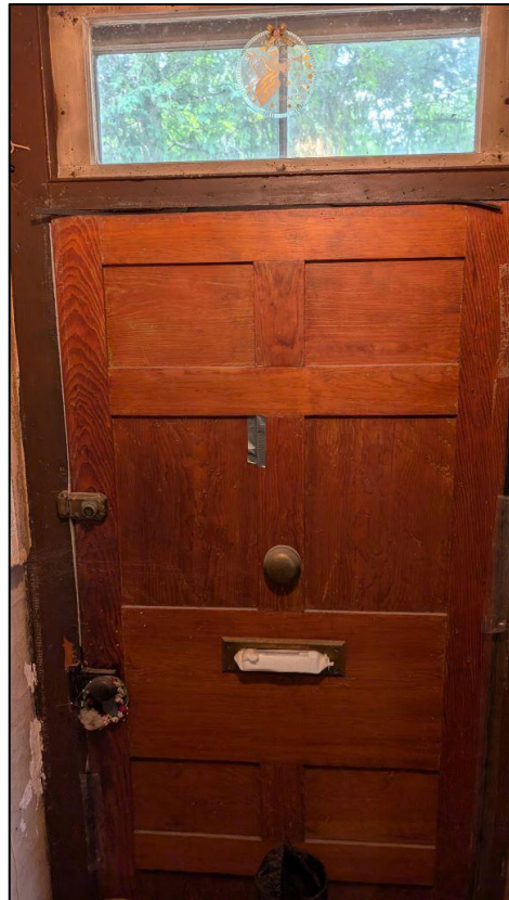
Figure 31: Wooden front door and transom found on the side (west) elevation of the existing dwelling (John Mark Rowe 2024)
