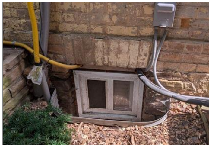
Figure 28: Basement windows on the extant dwelling (John Mark Rowe 2024)
