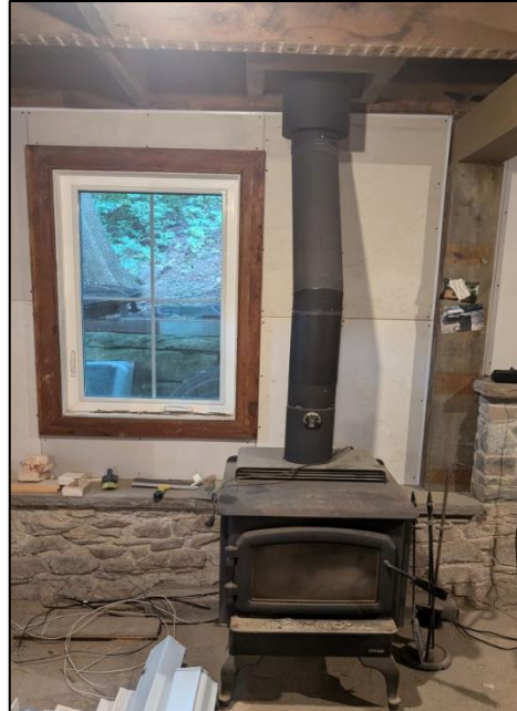
Figure 38: Existing fireplace in the extant dwelling (John Mark Rowe 2024)
