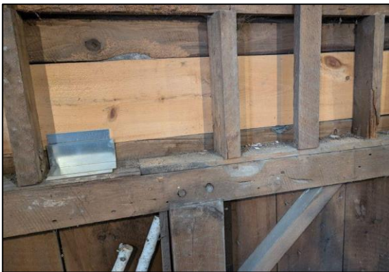
Figure 35: Interior of the framed summer kitchen (John Mark Rowe 2024)
