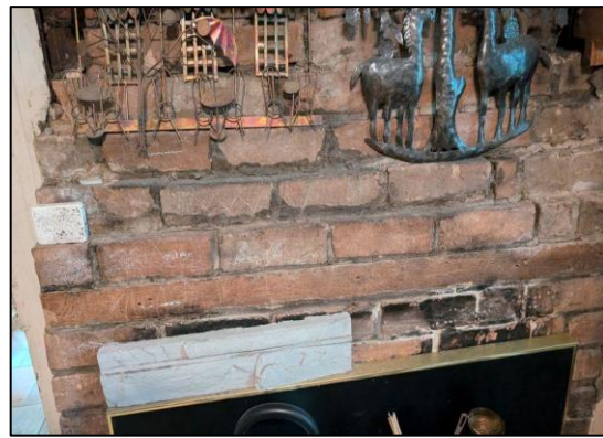
Figure 36: Existing fireplace in the extant dwelling (John Mark Rowe 2024)
