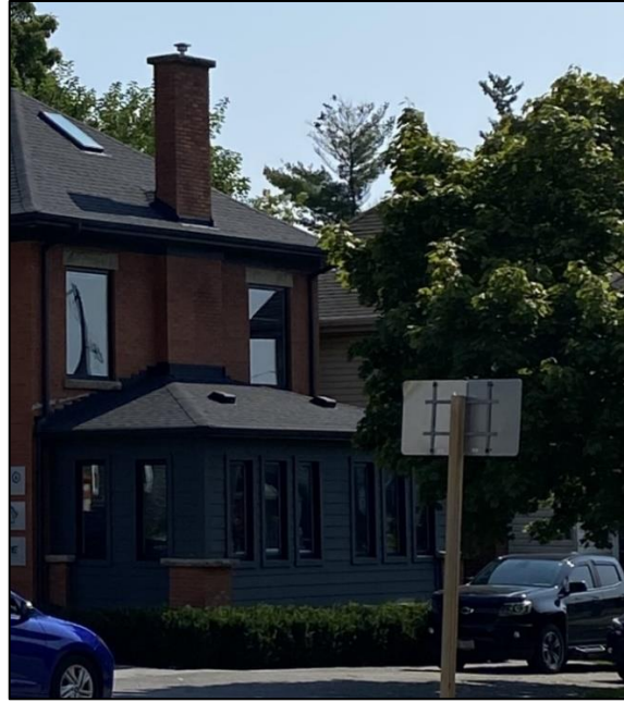
Figure 35: Side (southwest) elevation of the subject building (Town of Halton Hills 2024)
