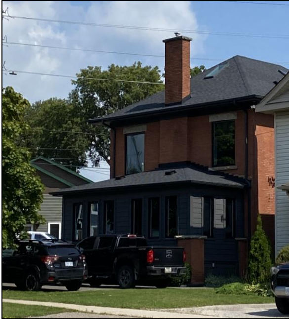
Figure 34: Side (southwest) elevation of the subject building (Town of Halton Hills 2024)
