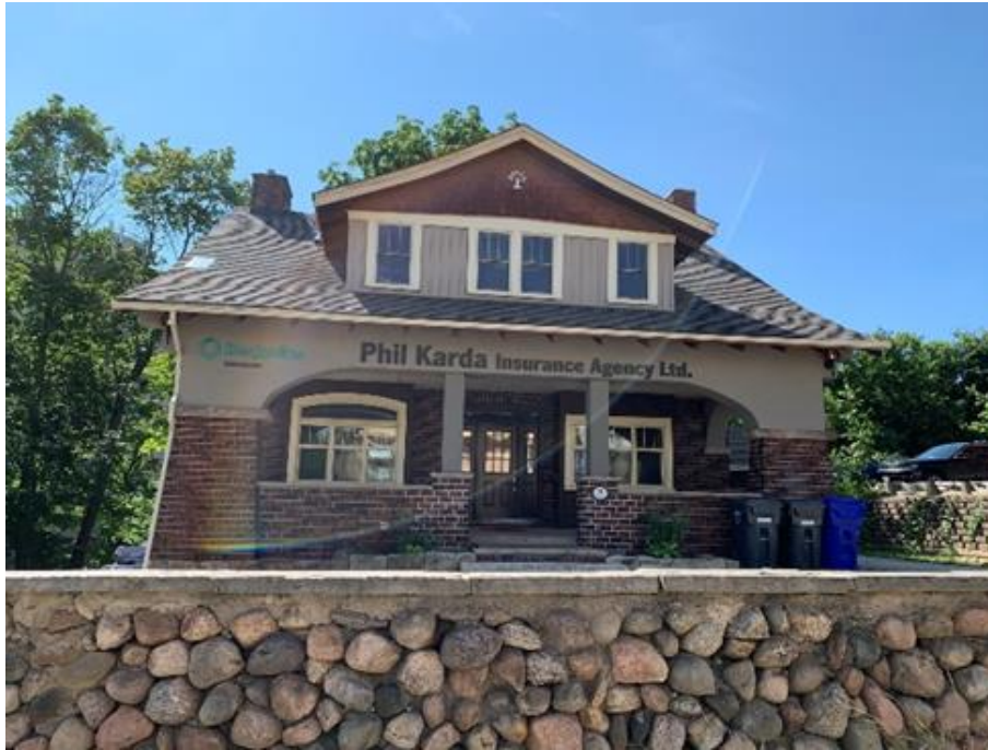
Figure 17: Front elevation of The Birches at 75 Mill Street, showing the cobblestone wall along Mill Street (Town of Halton Hills 2023)
