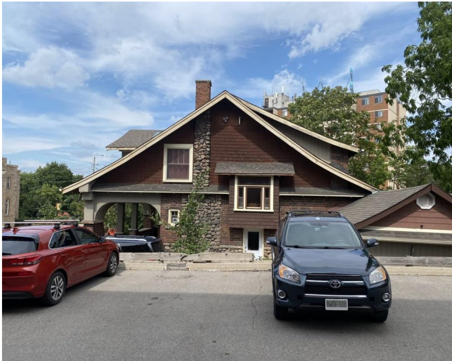
Figure 18: Southwest elevation of The Birches (Town of Halton Hills 2023)
