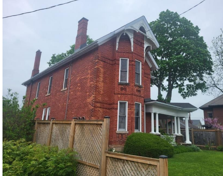
Figure 25: Northwest corner of the existing building at 39 Willow Street North (Town of Halton Hills 2024)
