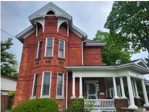
Figure 20: Front (west) elevation of the existing building at 39 Willow Street North (Town of Halton Hills 2024)
