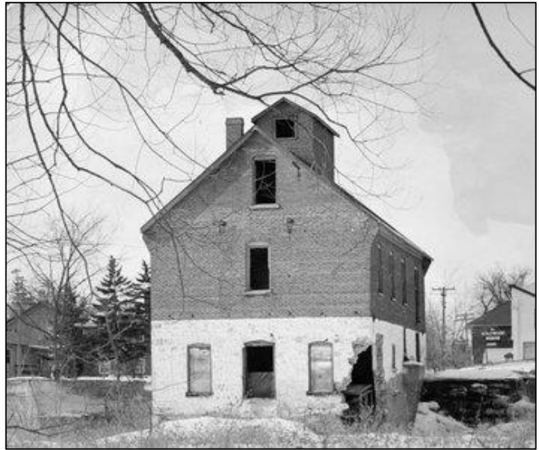
Figure 11: Image of the former Norval Flour Mills, prior to demolition c.1961 (EHS02326)
