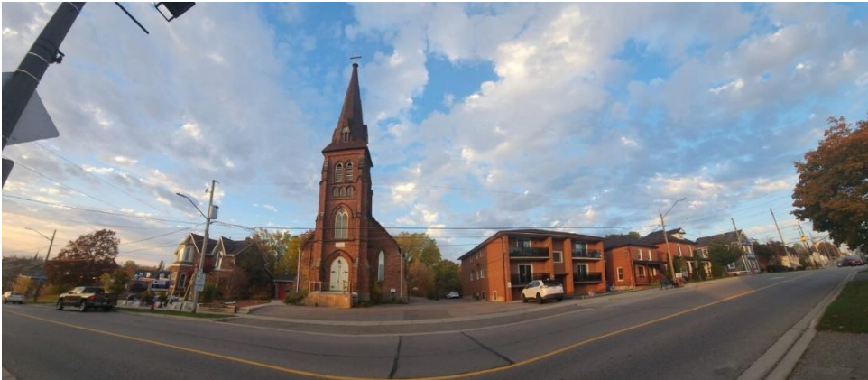
Figure 29: Panoramic view of the subject property along Main Street South (Town of Halton Hills 2023)
