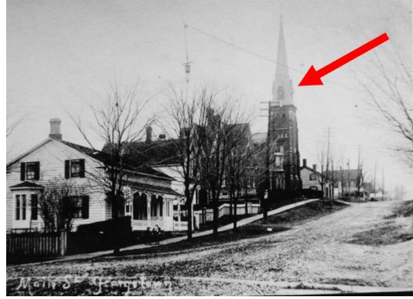
Figure 9: Intersection of Main and James Streets, Baptist Chapel identified in the background, c.1908 (EHS 11635)
