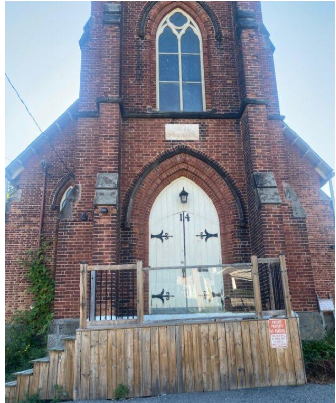
Figure 31: Detail of front (northeast) elevation of First Baptist Church at 14 Main Street South (Town of Halton Hills 2023)
