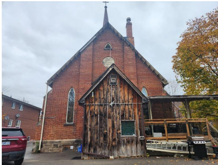
Figure 37: Rear elevation of First Baptist Church with one-storey frame addition (Town of Halton Hills 2023)
