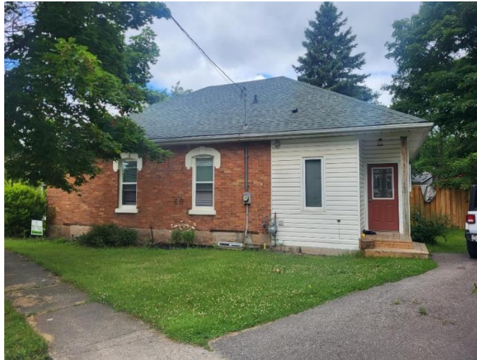
Figure 11: 23 Young Street, Side (East Elevation) (Town of Halton Hills 2024)
