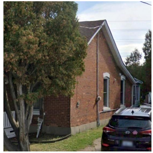
Figure 16: Side Elevation of 58 Young Street featuring segmentally arched windows. (Google Street View, 2023)
