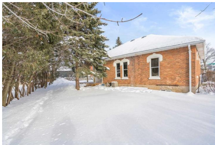
Figure 12: 23 Young Street, Side (West) Elevation (House Sigma 2023)
