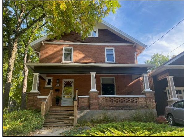
Figure 26: Front (northwest) elevation of the existing dwelling (Town of Halton Hills 2023)
