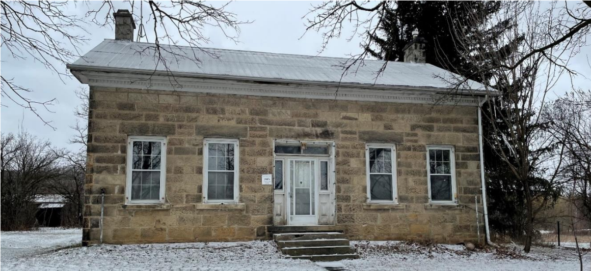
Figure 22: Front (southeast) elevation of the Duncan McCallum House (Town of Halton Hills 2024)
