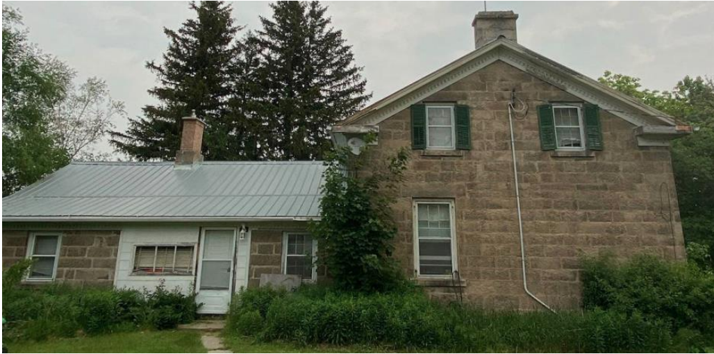
Figure 24: Side (southwest) elevation of the Duncan McCallum House (Courtesy Avison Young)
